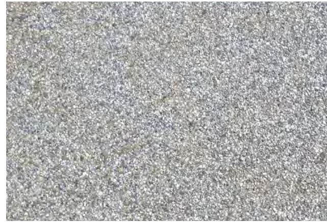
Exposed Aggregate Concrete Pavement
