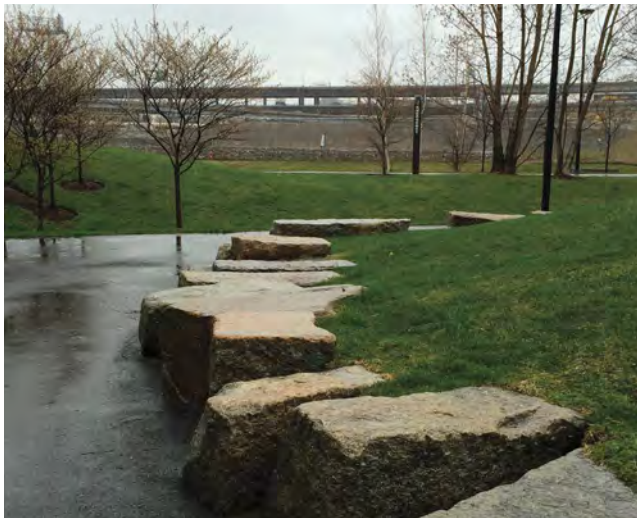
Reclaimed Granite Block Seatwalls
