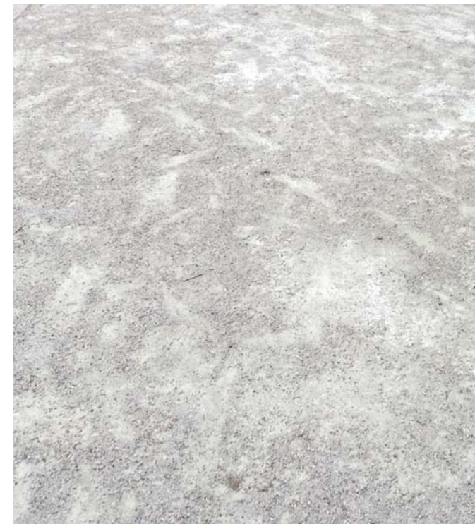
Decomposed Granite Pavement
