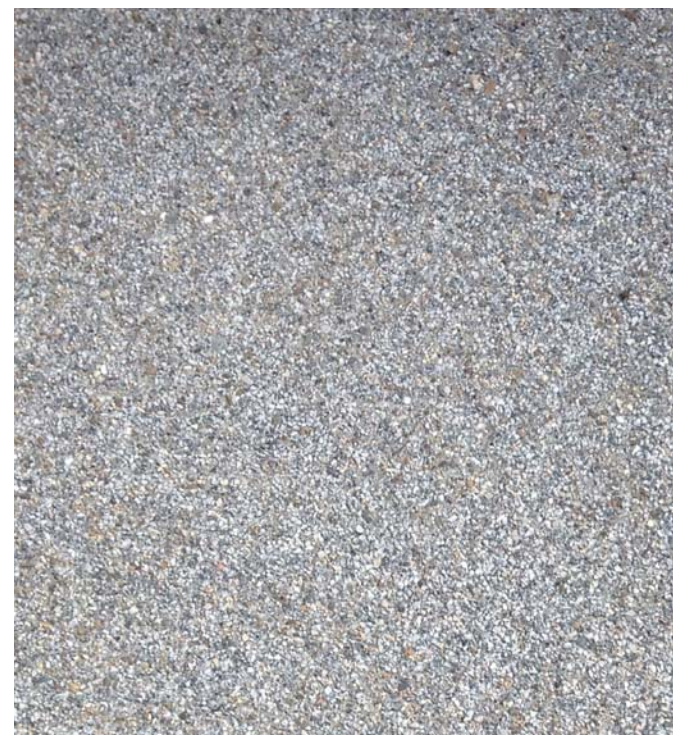
Exposed Aggregate Concrete Pavement
