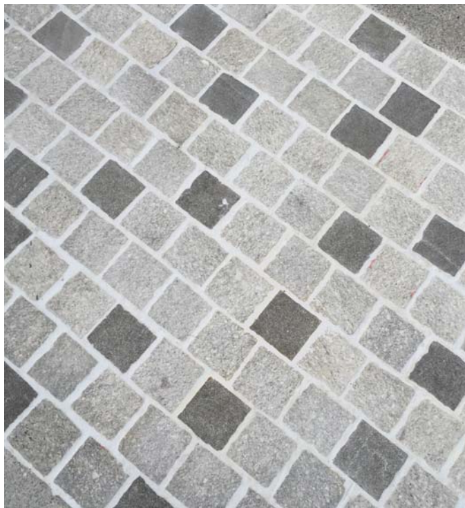
Stone Setts Pavement
