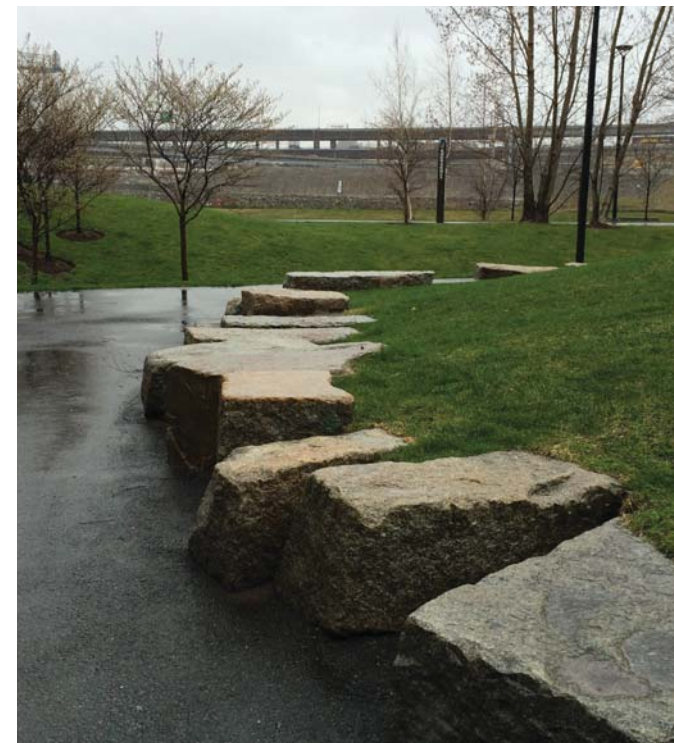
Reclaimed Granite Block Seatwall
