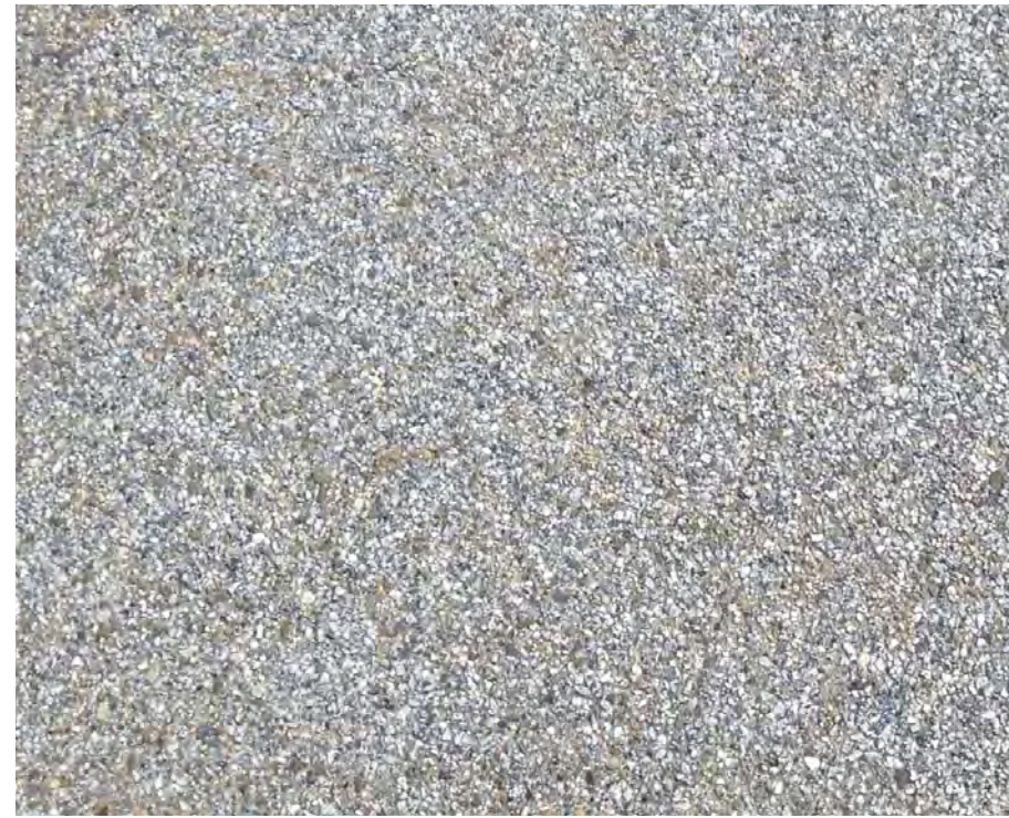
Exposed Aggregate Concrete Pavement
