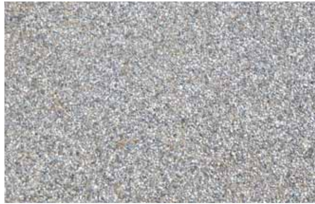
Exposed Aggregate Concrete Pavement
