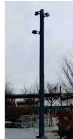
Light Pole - Morgan Ave
