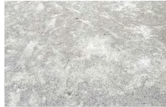
Decomposed Granite Pavement
