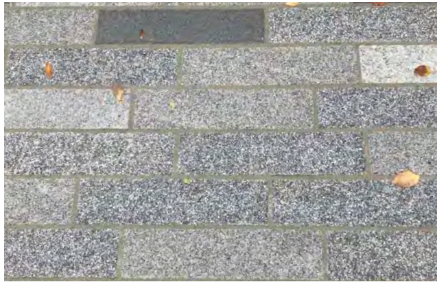
Stone Setts Pavement
