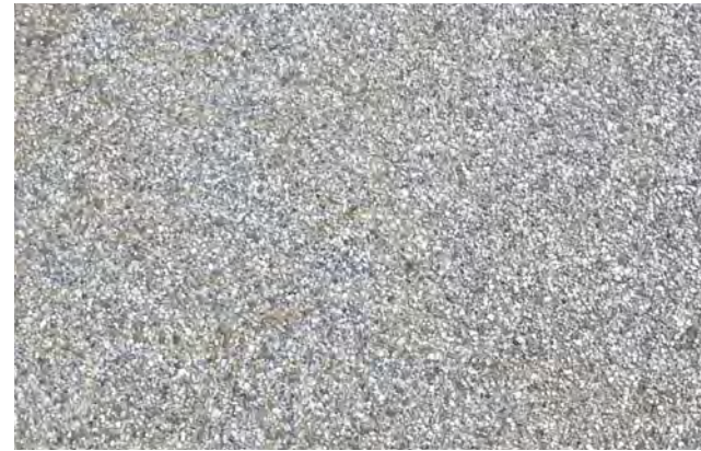
Exposed Aggregate Concrete Pavement
