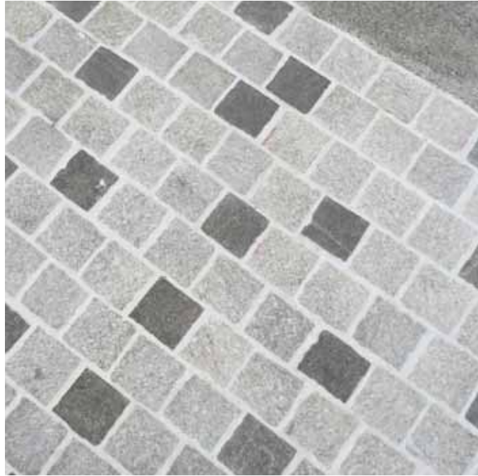
Granite Setts Pavement
