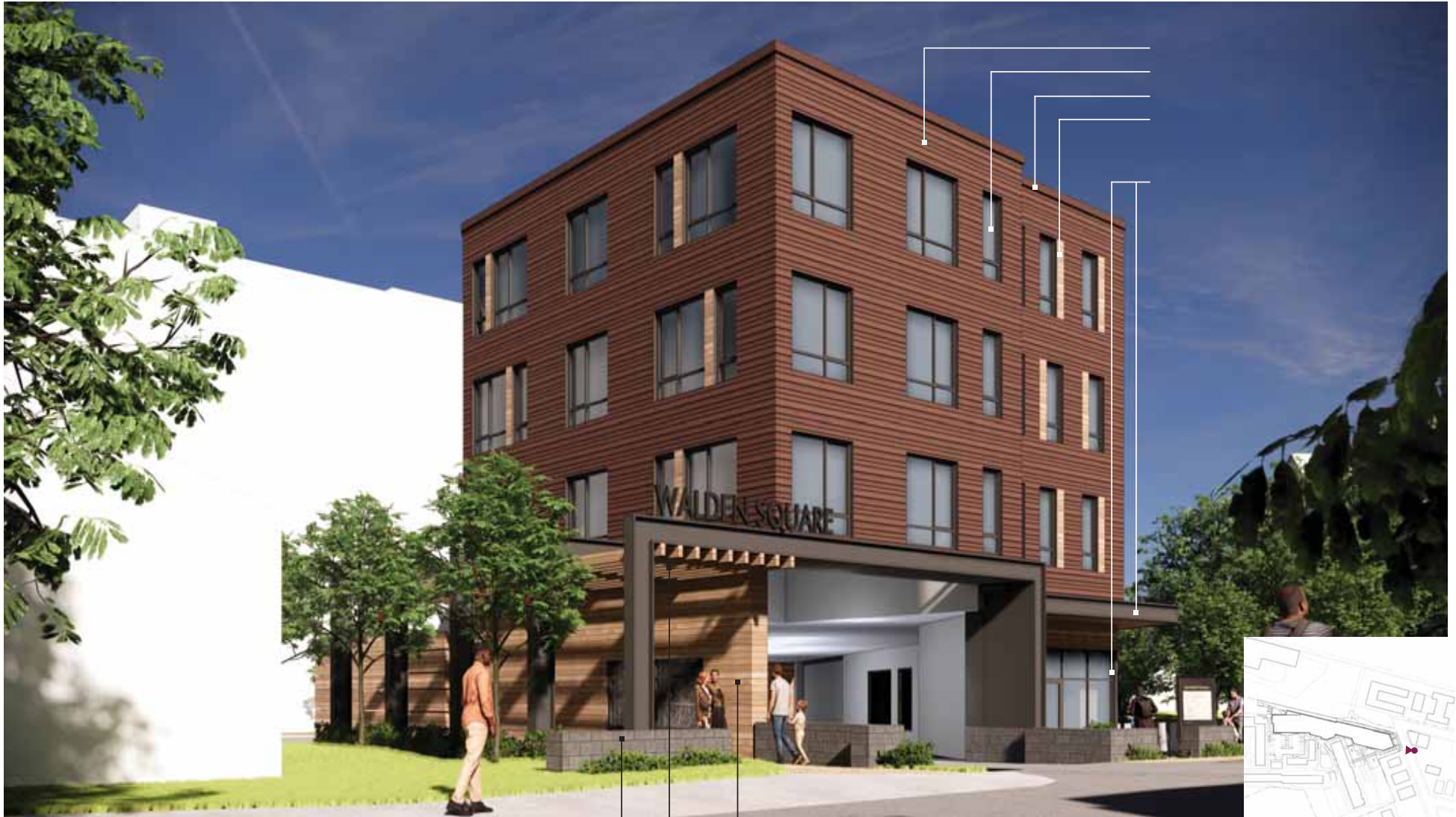
LOW CMU WALLS SEPARATE PEDESTRIANS FROM VEHICLES
