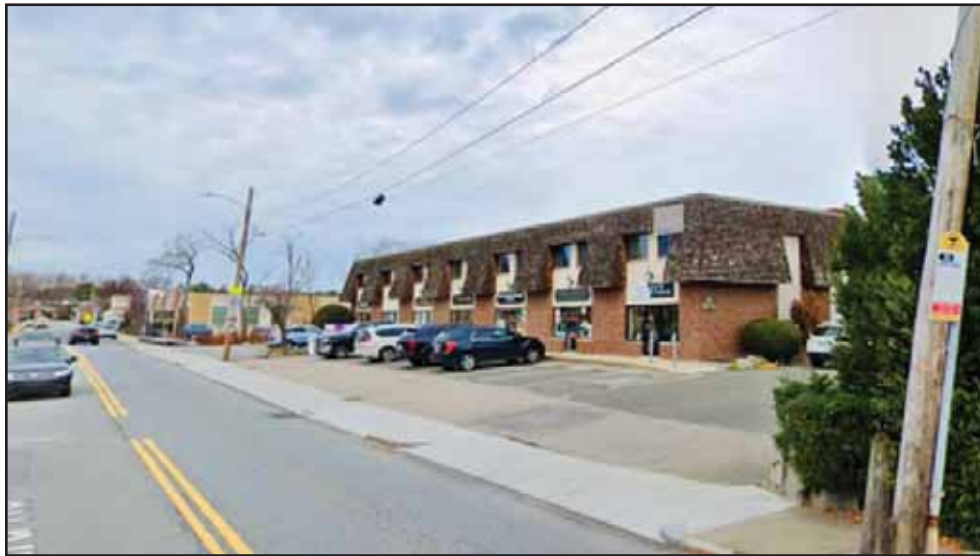
Photo of Existing Building Looking North
