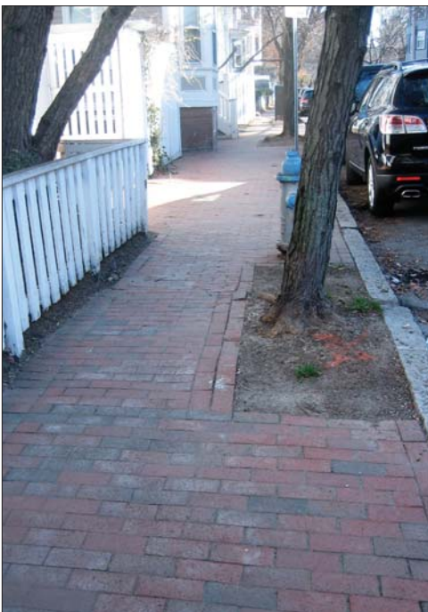
Figure 18. Re-bricked sidewalk on Franklin Street in Riverside, with brick set on sand over an asphalt base.
