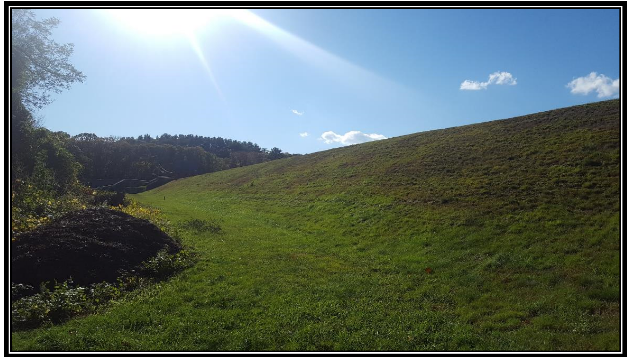
Downstream slope of Stony Brook Dam, 10/31/2017
