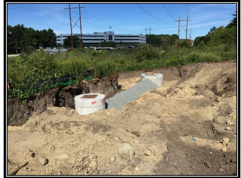
8/30/2016 inspection at 200 Smith St Waltham
