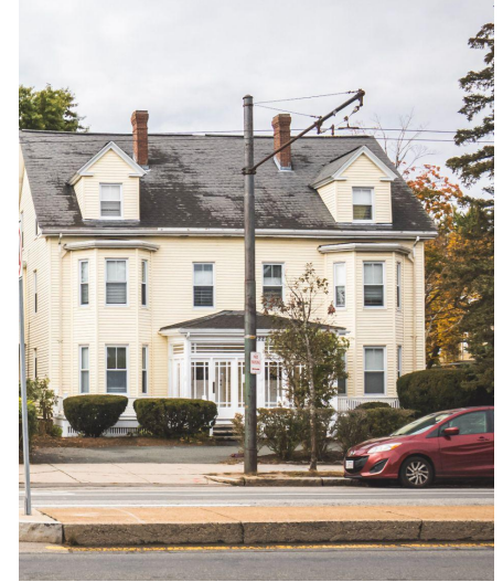
Legacy streetcar trolley infrastructure still remains, but is being removed.
