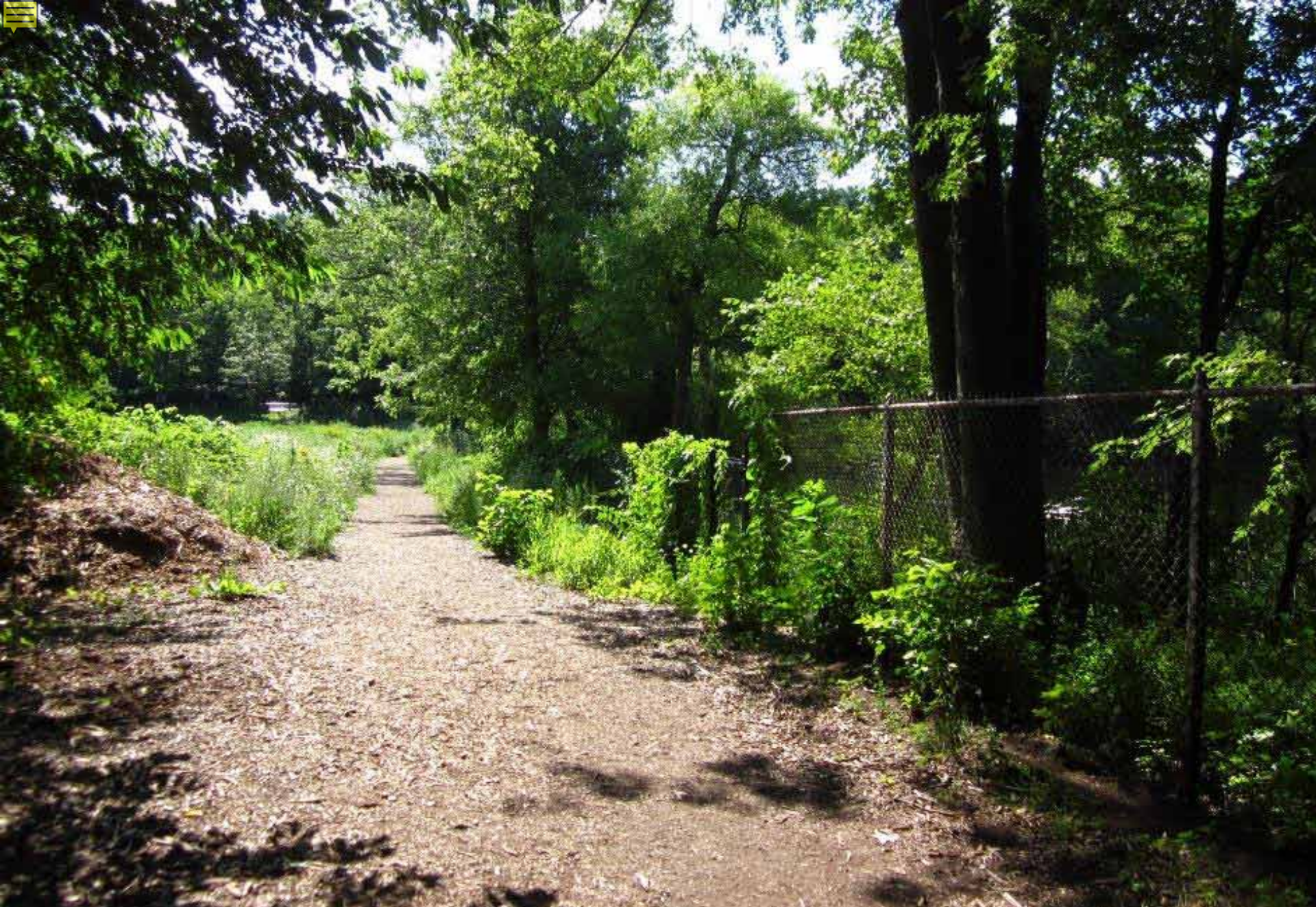
BASE LOOP TRAIL – MULCH (NON-COMPLIANT)
