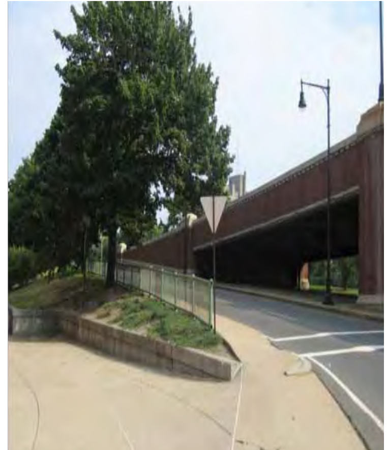
Pedestrian circulation around bridges needs improvement.
