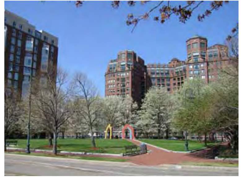
Front Park with the Esplanade housing on the left and the River Court housing in the background.
