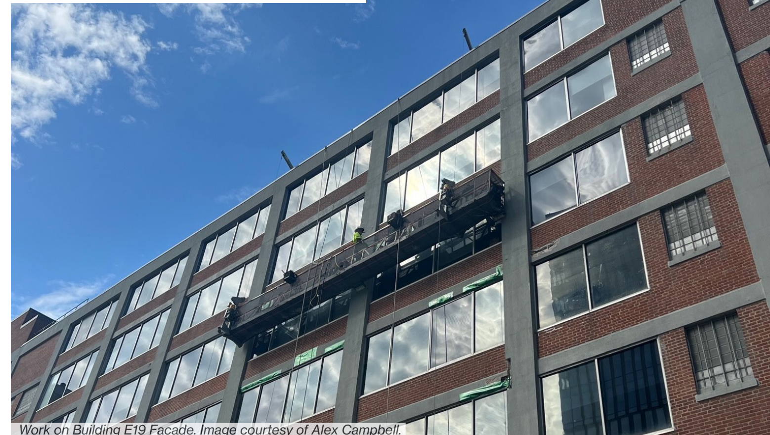
Work on Building E19 Façade. Image courtesy of Alex Campbell.
