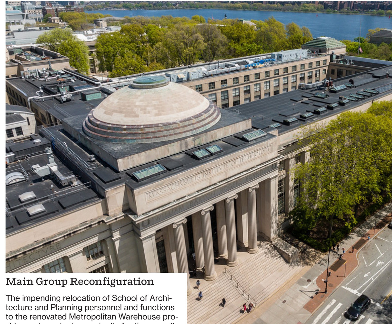
Aerial view of Building 7. Image courtesy of Emily Dahl.
