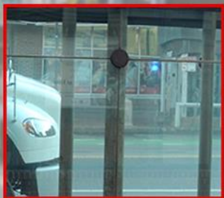
GLAZING AT ESCALATOR HEADHOUSE
