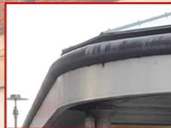
ESCALATOR HEADHOUSE ROOF
