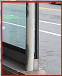
METAL TUBE AS COLUMNS
