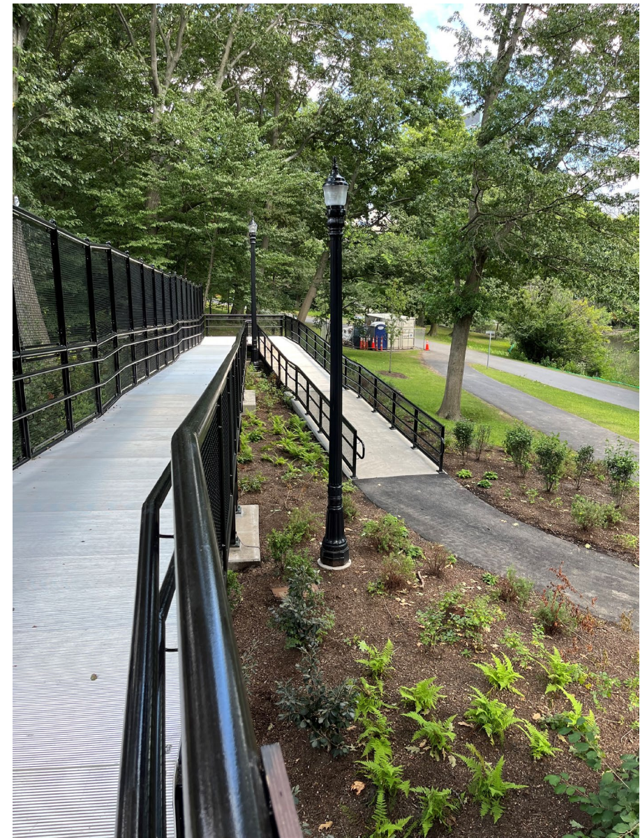
Carlton Street Footbridge Brookline, MA
