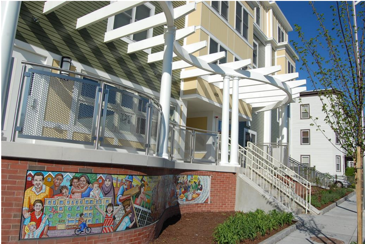
Putnam Green Apartments: 40-unit affordable development approved by a special permit by the Planning Board
