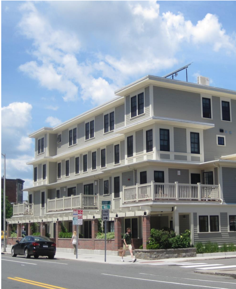
Main and Cherry Condos: 10 affordable units approved by comprehensive permit
