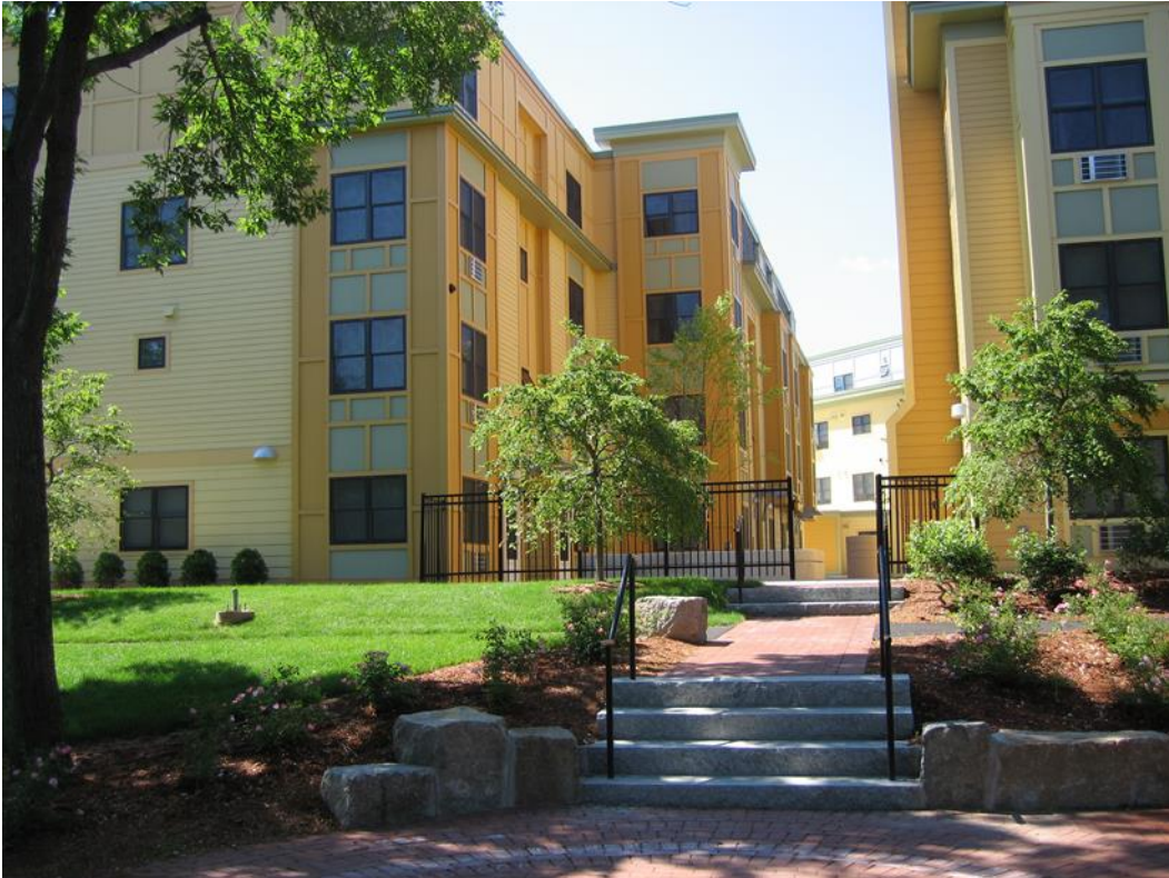
Trolley Square: new construction of 40 affordable units in mixed-use development
