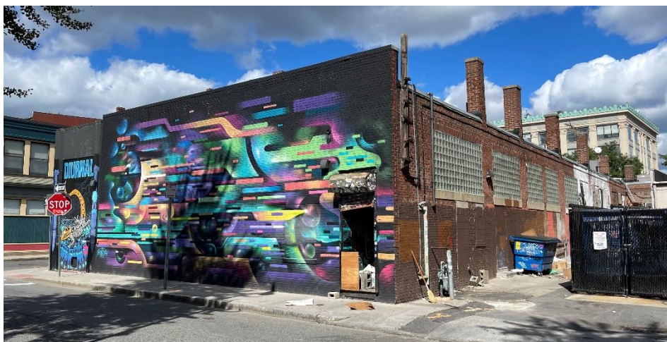
2-10 Brookline Street/468-480 Mass. Ave., Green Street (left) and rear façade (right).
