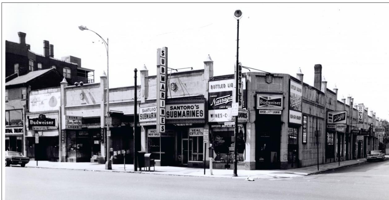
468-480 Massachusetts Avenue showing parapet and storefront detail before renovations. CHC photograph taken July 1969.
