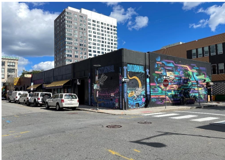
2-10 Brookline Street/468-480 Mass. Ave., Brookline Street (left) and Green Street façades.
