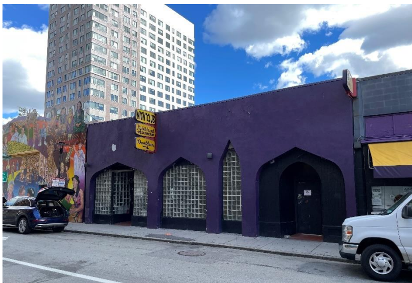
Original Middle East Restaurant entrance on Brookline Street. Ogee arched openings and glass block windows as part of likely 1980 renovation.
