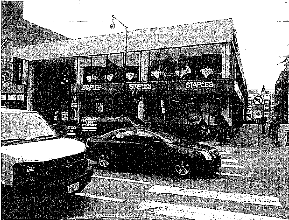
Fig 1- View of the building from the N.E. corner of JFK and Winthrop St.
