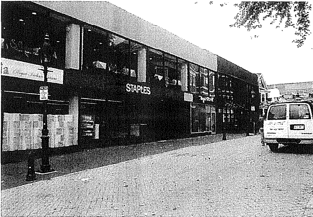
Fig 3 – View of the proposed space from JFK Street.
