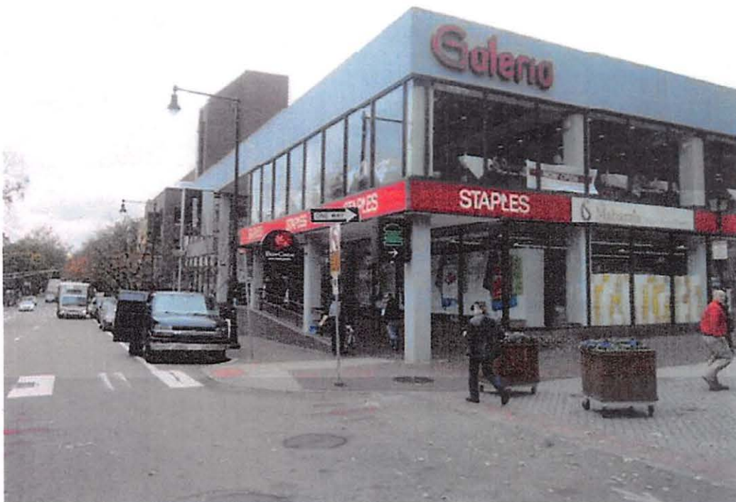
Fig 2 – View of N.E. corner of building
