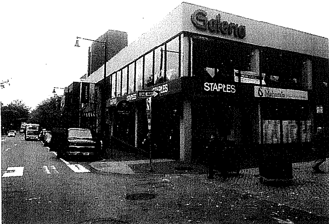
Fig 2 – View of N.E. corner of building
