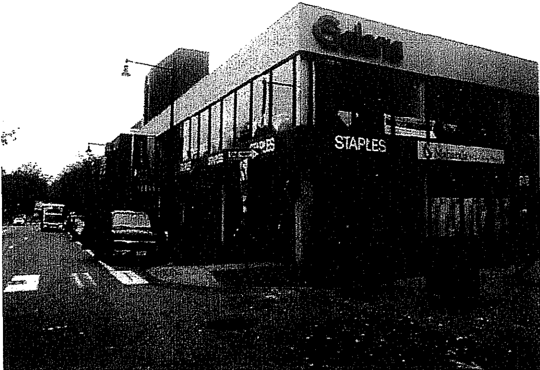
Fig 2 – View of N.E. corner of building
