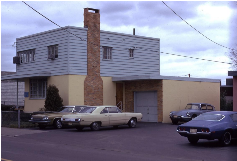
47-53 Bay State Road, 1974. Photograph taken prior to 1979 two-story addition. Image courtesy of Sky & Telescope Magazine .
