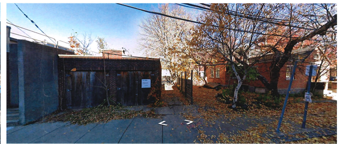
GARAGE FROM BENT STREET
