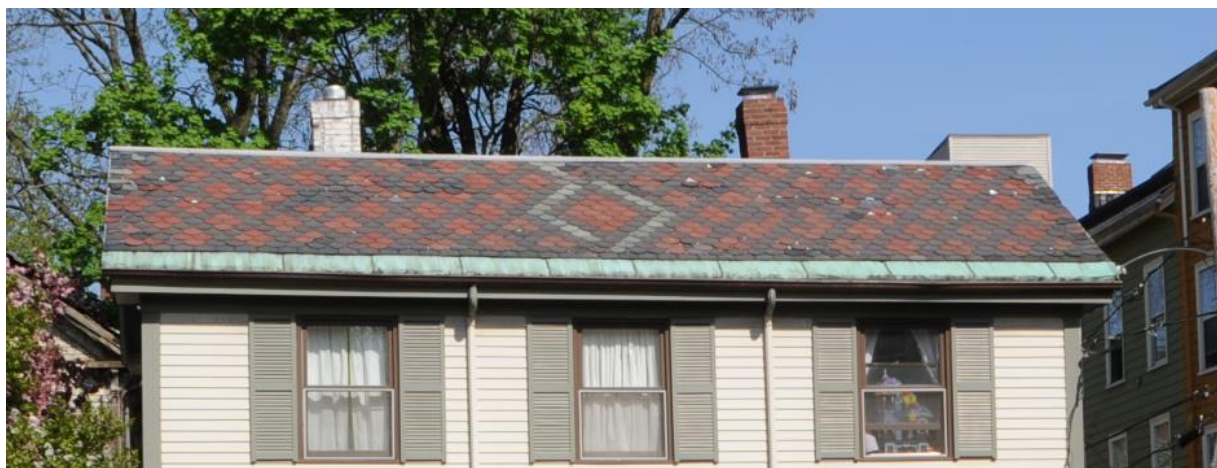
48 Banks Street slate detail, CHC photo 2015.
