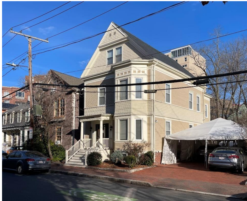
38-40 Banks Street façade and south elevation.
