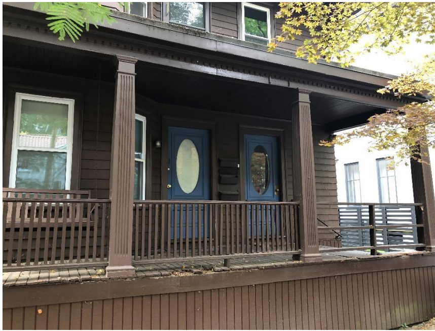
68-70 Lexington Avenue, front porch and door detail. CHC photo, 2020.
