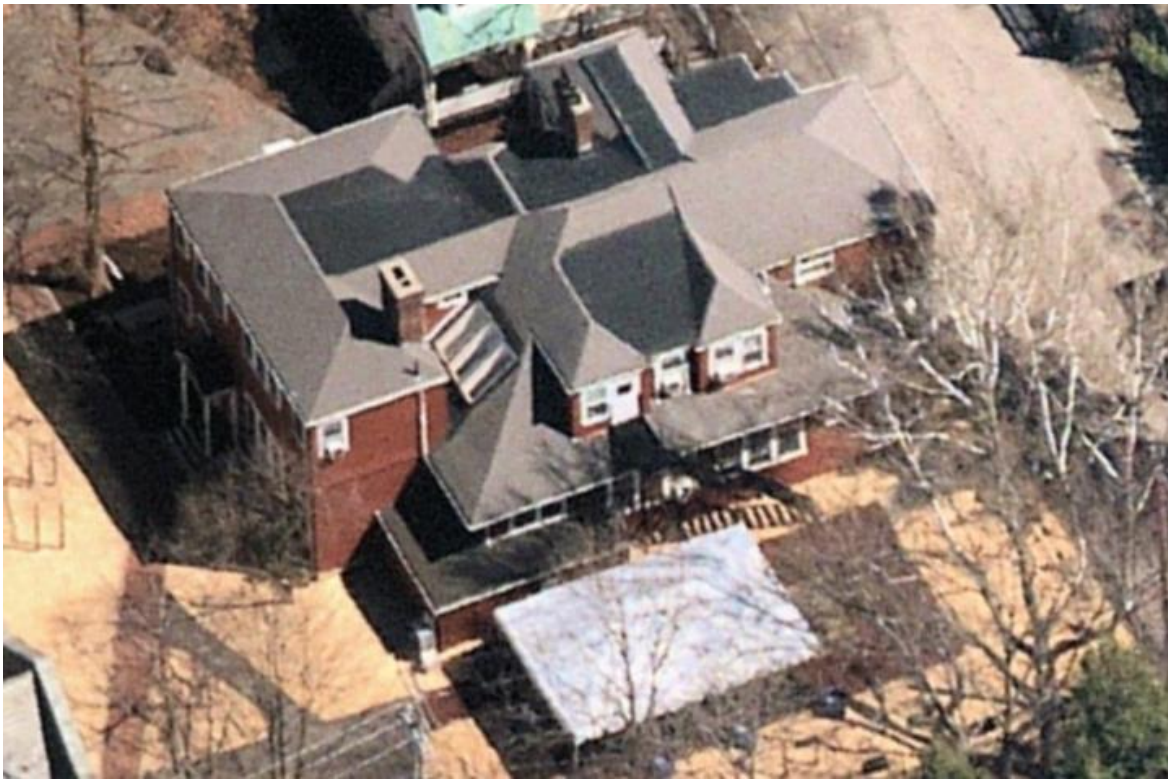
Aerial view of the Markham building, 27 March 2021. From Nearmap.com, accessed 5 Nov. 2021.
