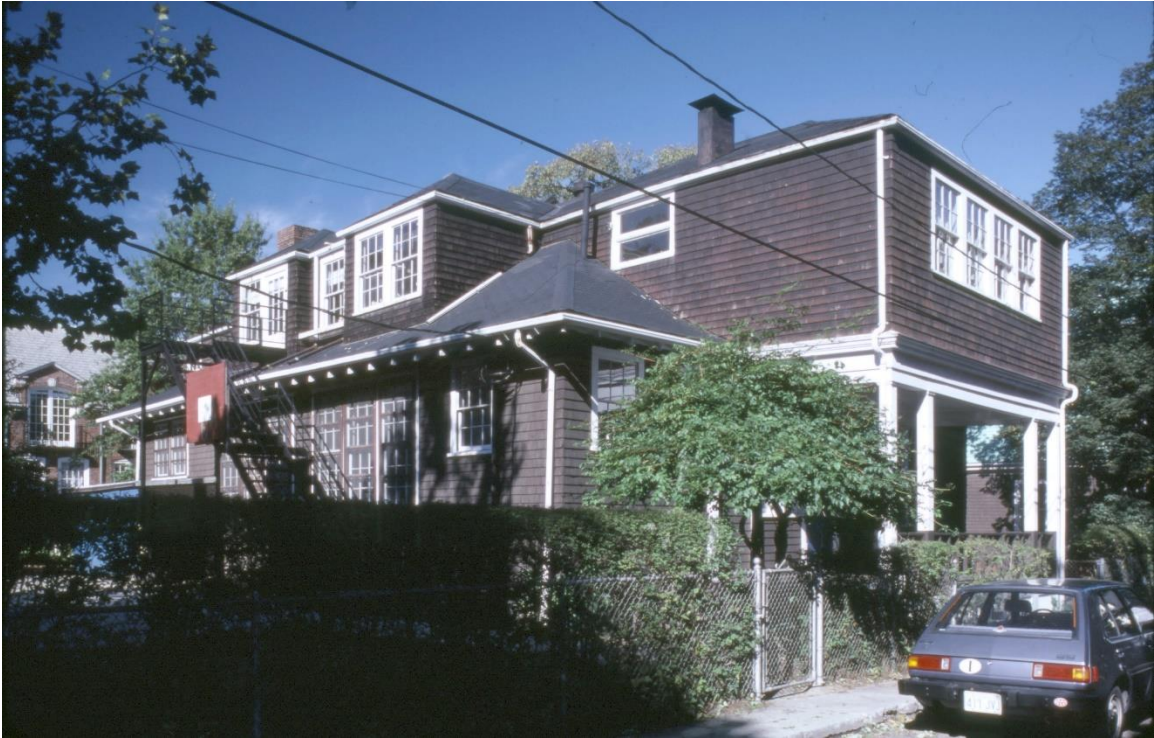
Markham Building from the southwest, 1983. Christopher Hale photo, CHC Collections
