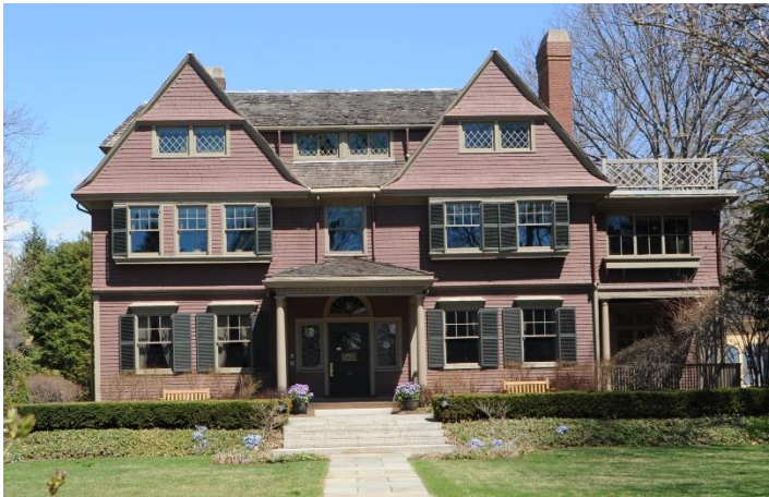
113 Brattle St. (1887, Andrews, Jaques & Rantoul, architects)
