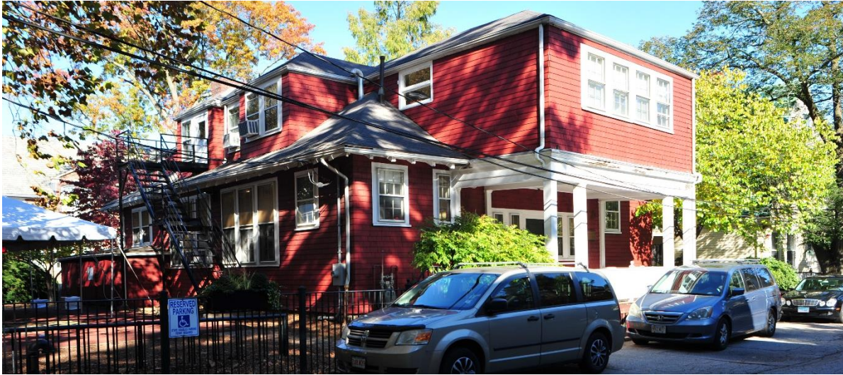
West and south elevations of the Markham building at 10 Buckingham St. CHC staff photo, Nov. 2021.
