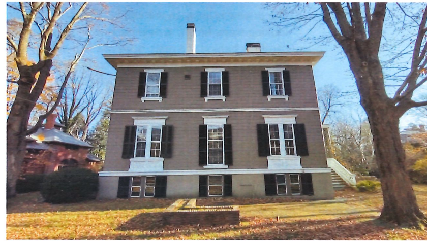
LEFT FACADE (FACING SPARKS STREET)
