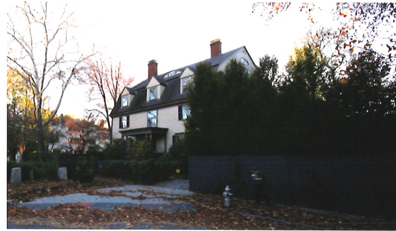
CURRENT VIEW FROM IRVING ST
