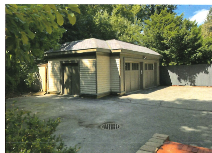
VIEW OF GARAGE LOOKING NORTHWEST
