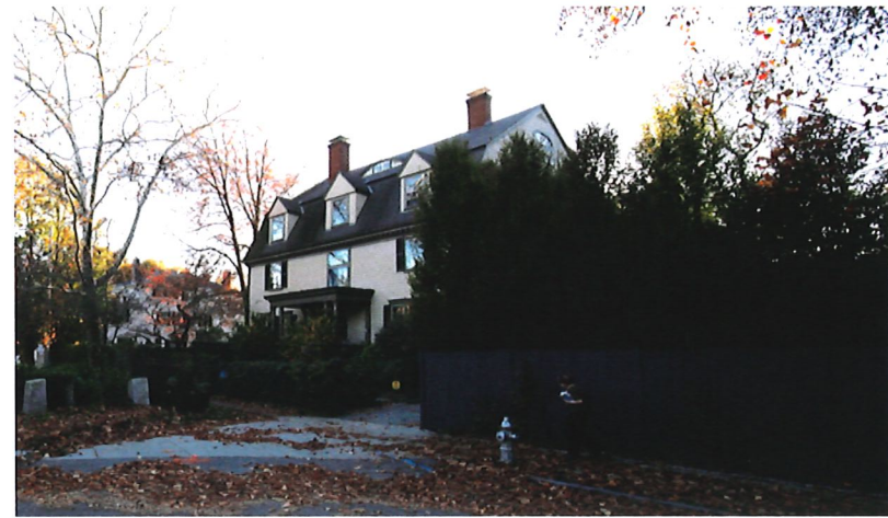
CURRENT VIEW FROM IRVING ST
