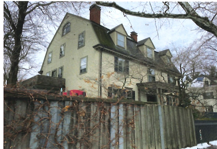
VIEW FROM SIDEWALK ON IRVING STREET LOOKING NORTHWEST
