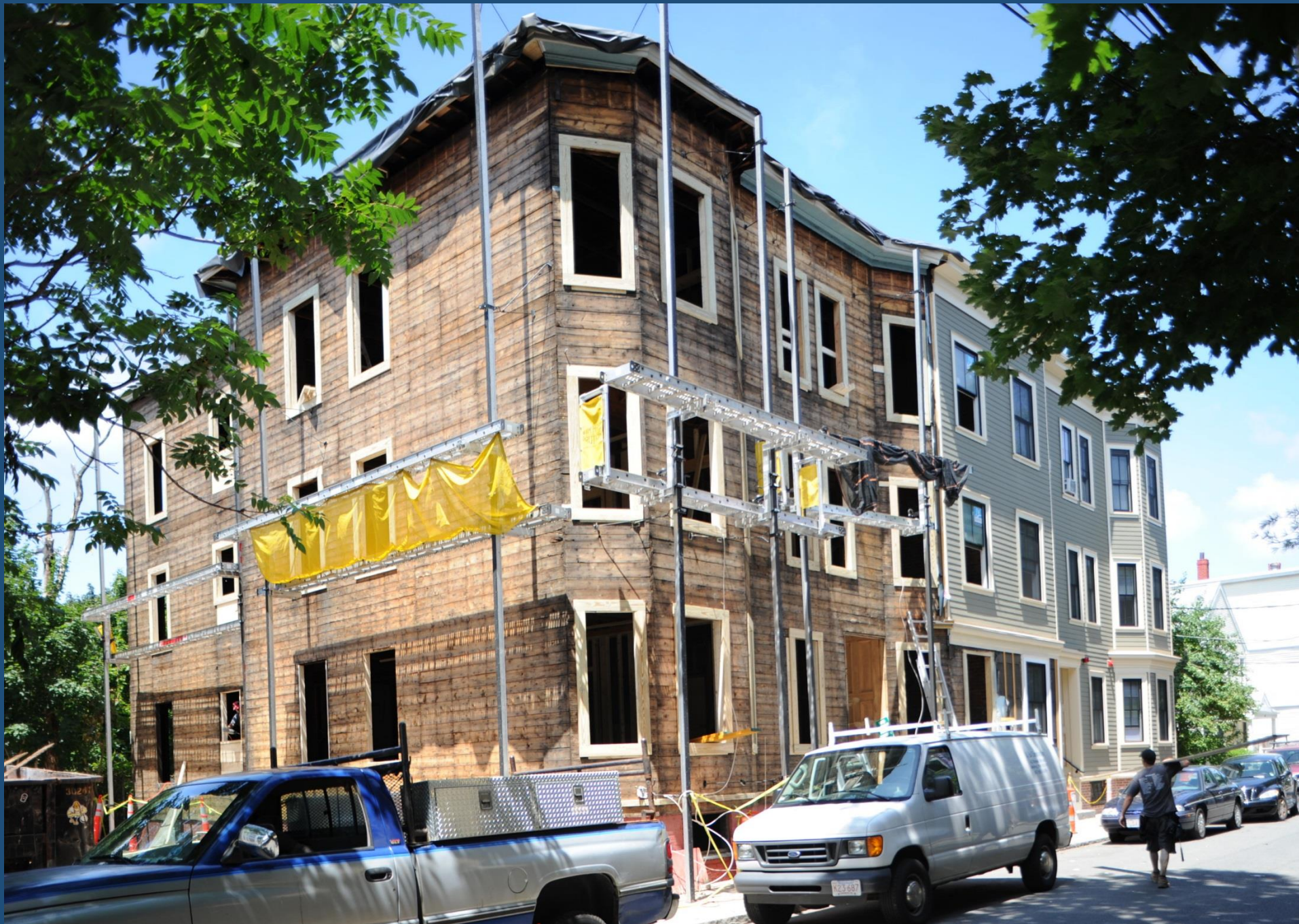
93-97 Pine Street, 1903 Agency-owned Rehabilitated 2010
