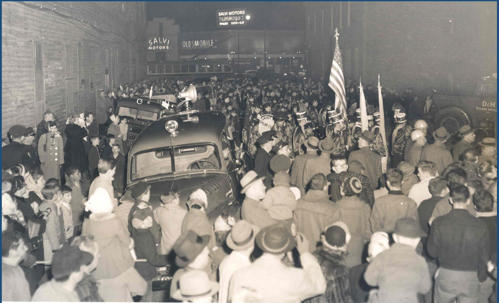
Demolition of the Rogers Block, 1957
