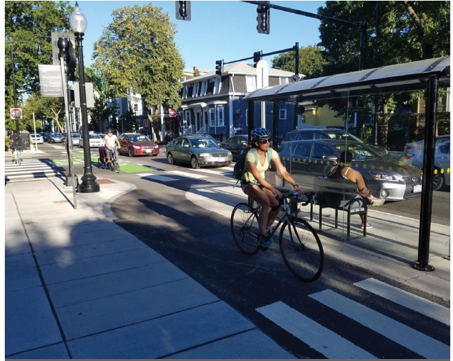
An example of a full construction bus boarding island with raised bike lane. (Recommended)
