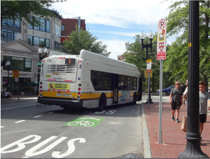
An example of a quick-build shared bike lane and bus stop. (Not Recommended)
