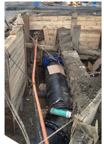
New 30-inch water main installed on Huron Ave
