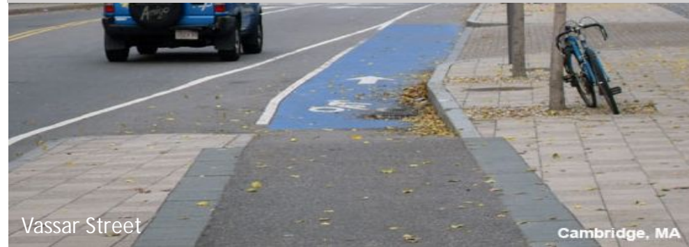
Bicycle Ramp: Sidewalk Level to Roadway Level The bike lane transitions from sidewalk level to roadway level before a horizontal transition.
