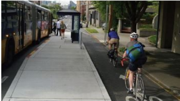
Floating bus stop with separated bike lane
