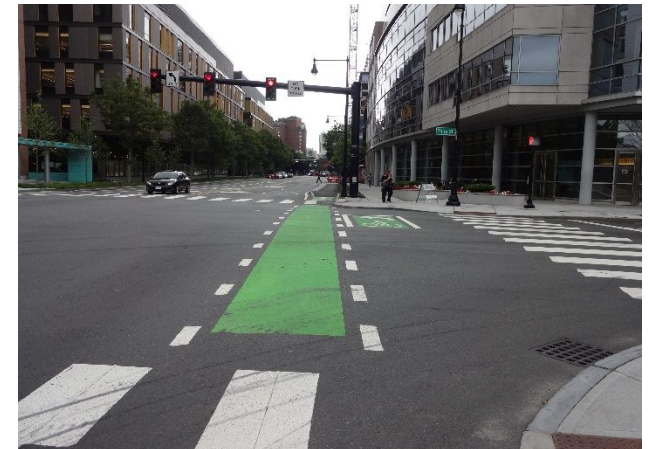
Colored pavement markings
