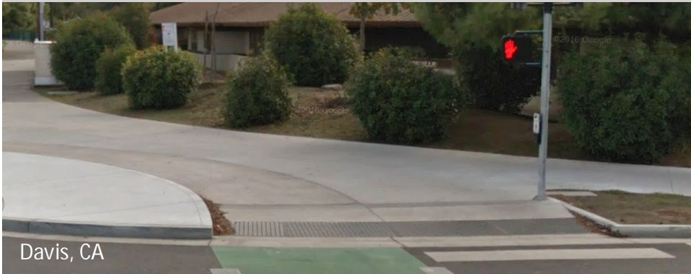
Shared Bike/Ped Crossing at Protected Intersection Bicycle and pedestrian areas are combined and lowered to create one short ramp. The ped/bike areas are delineated with colors.
