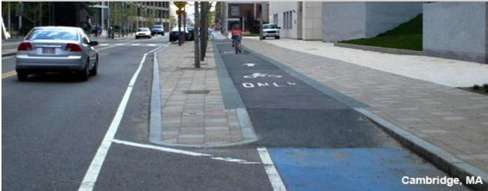
Bicycle Ramp: Roadway Level to Sidewalk Level The bike lane transitions to sidewalk level without a horizontal transition.
