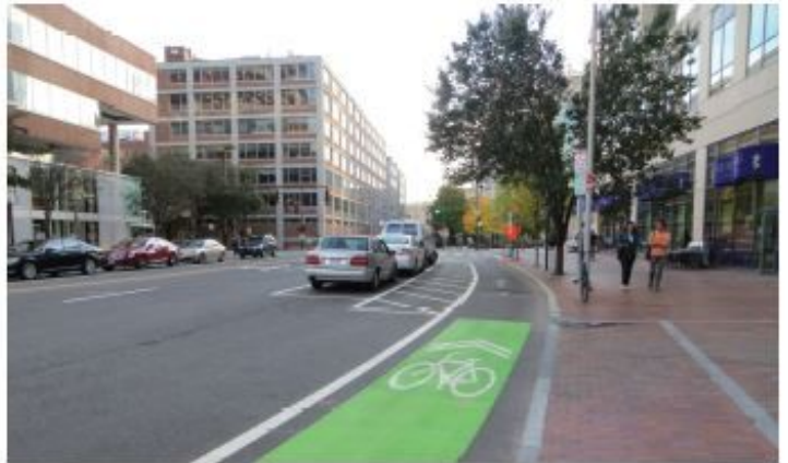
Colored pavement markings
