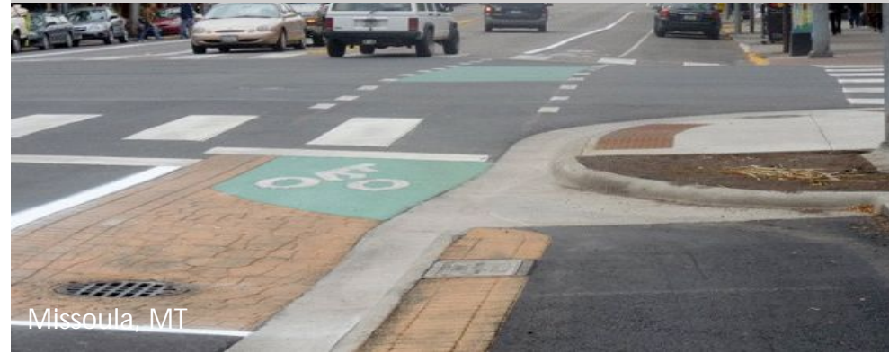
Bicycle Ramp: Sidewalk Level to Roadway Level Transitions both vertically and horizontally from sidewalk level to roadway level. Uses a "Bend-Out" intersection treatment.
