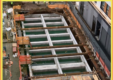
The Parking Lot 6 Tank constructed during Phase 1.
