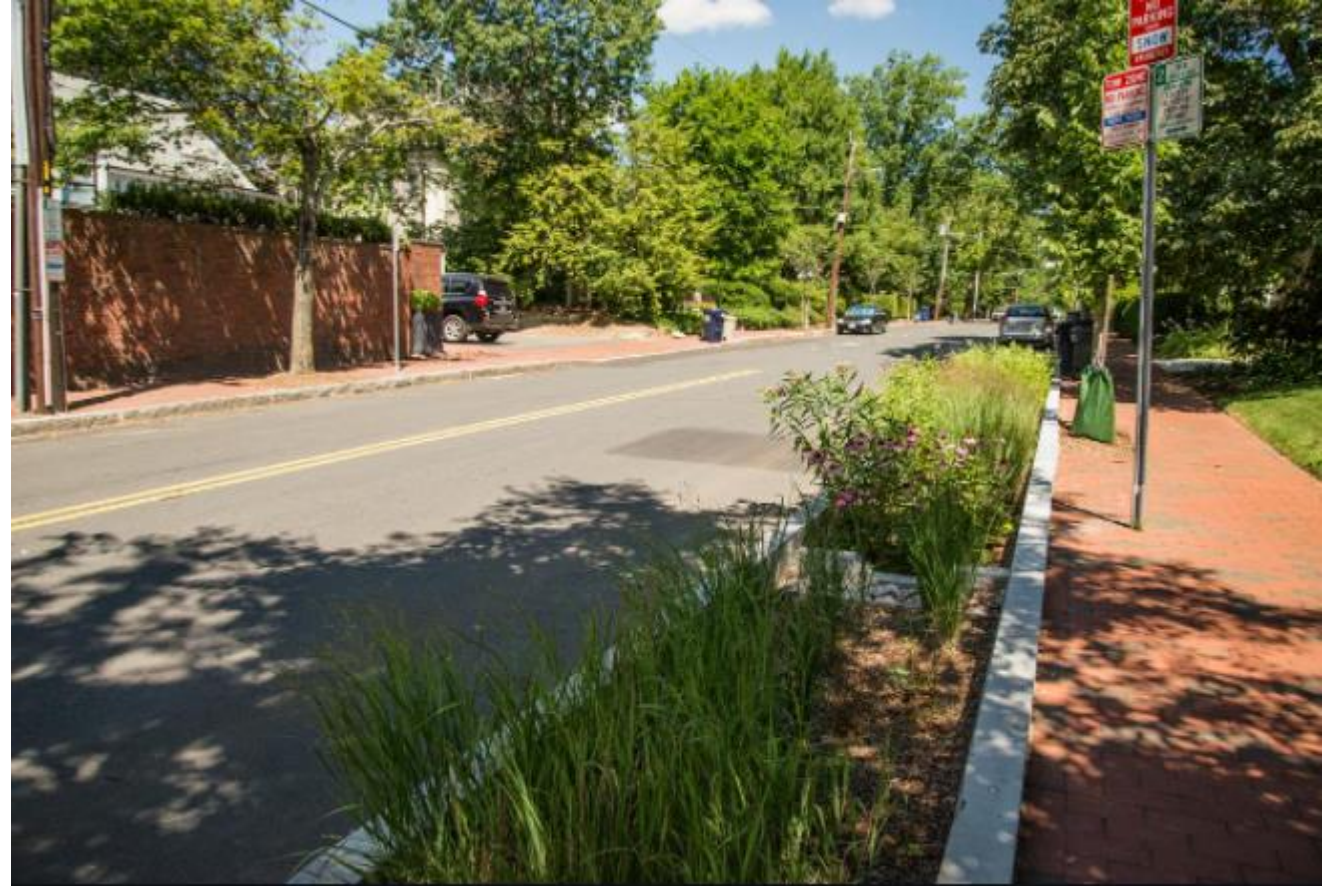
Existing green infrastructure biobasin on Lakeview Avenue.
