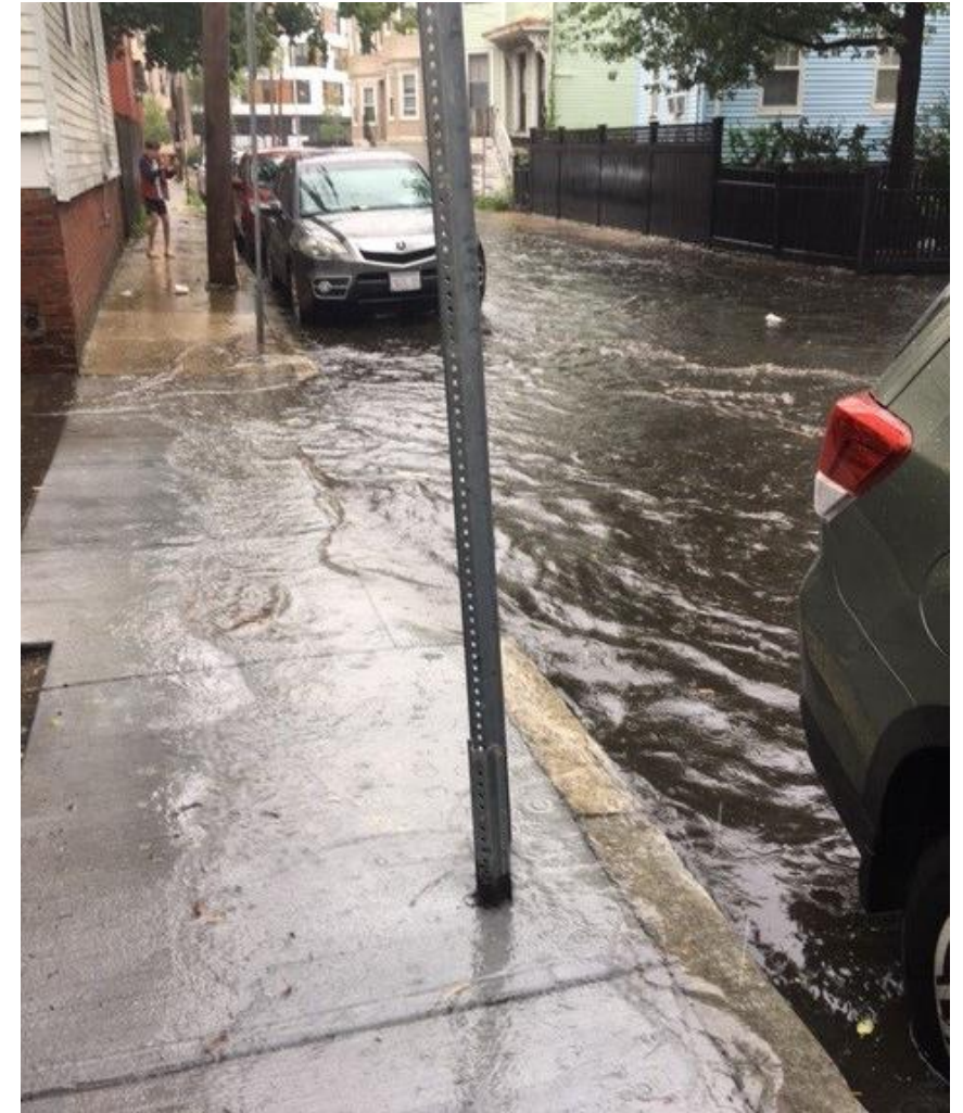
Stormwater flooding on School Street from a storm on August 19, 2021. Photo by Randa Ghattas
