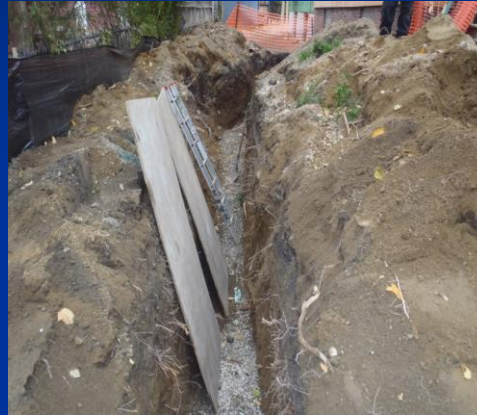
Inadequate support
