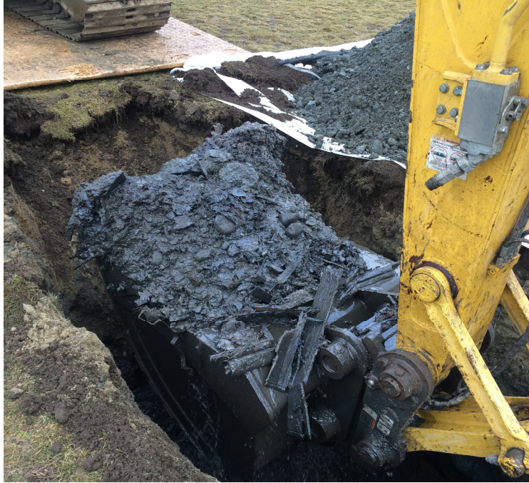
-Bucket of waste fill material from approximately 12' bgs.
