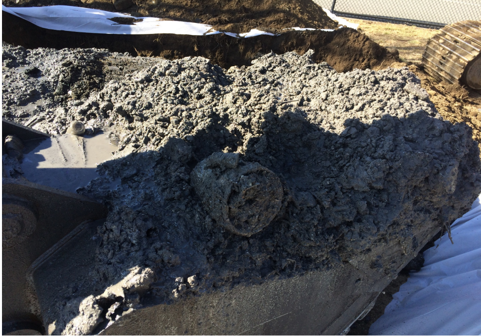
-Bucket of waste fill material from approximately 15' bgs
