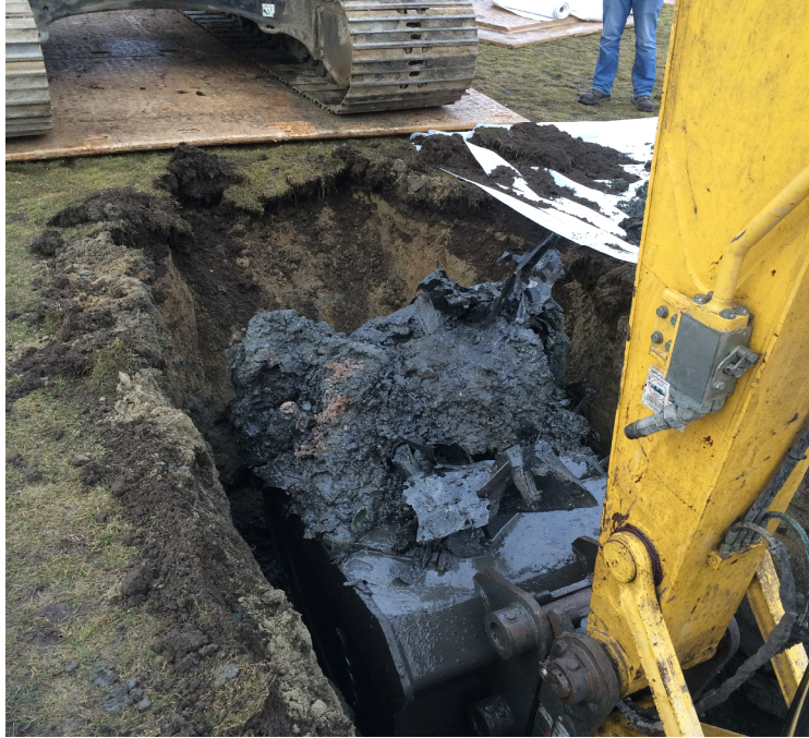
-Bucket of waste fill material from approximately 10' bgs.
