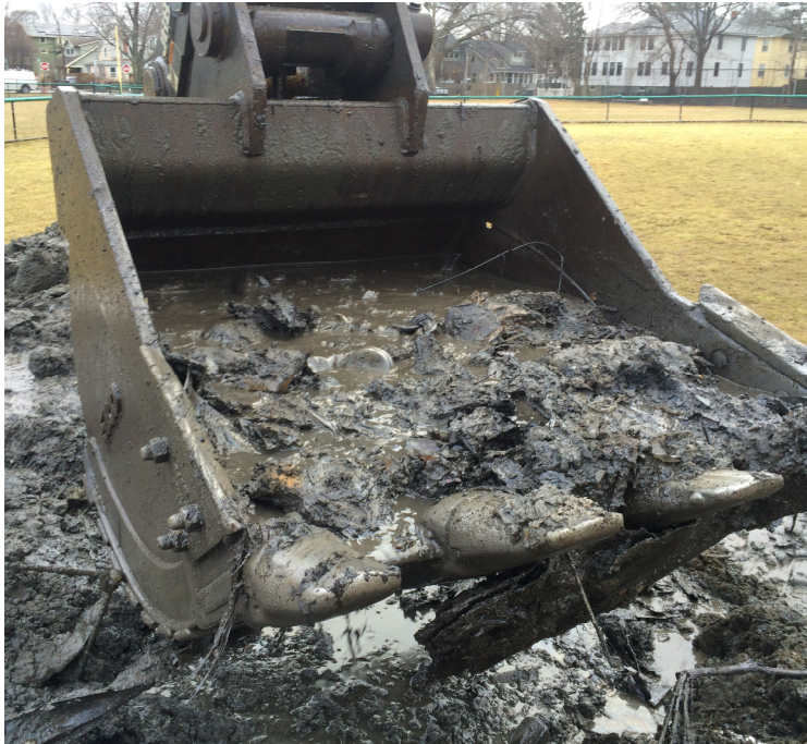
-Bucket of waste fill material from approximately 15' bgs.
