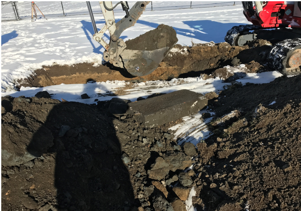
-Stockpile of waste fill material showing granite block from approximately 5' bgs
