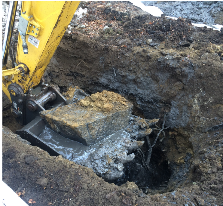
-Bucket of waste fill material from approximately 9' bgs.
