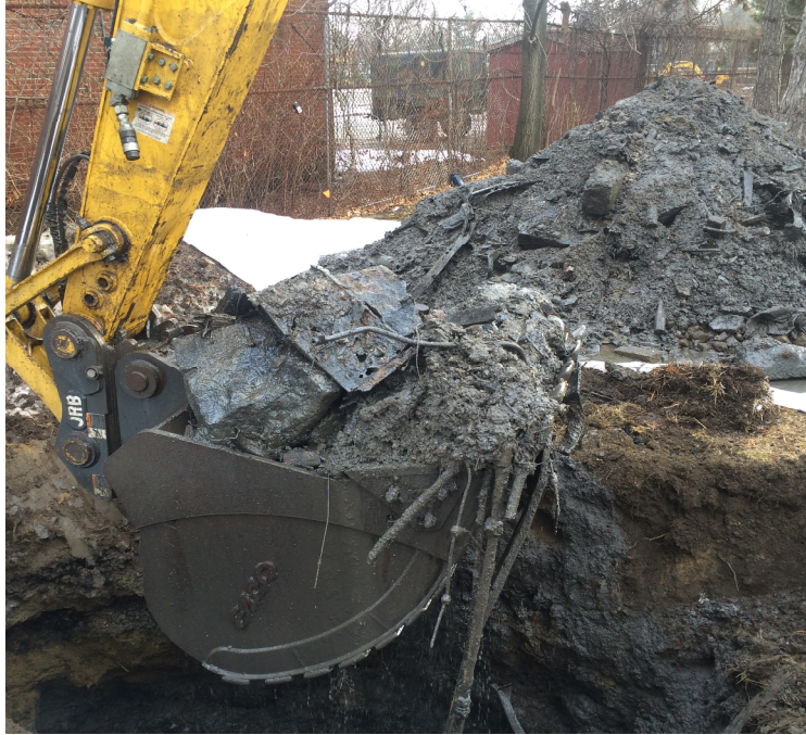
-Bucket of waste fill material from approximately 13' bgs.
