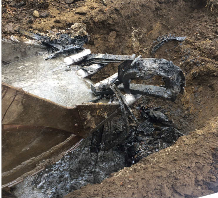
-Bucket of waste fill material from approximately 8' bgs.
