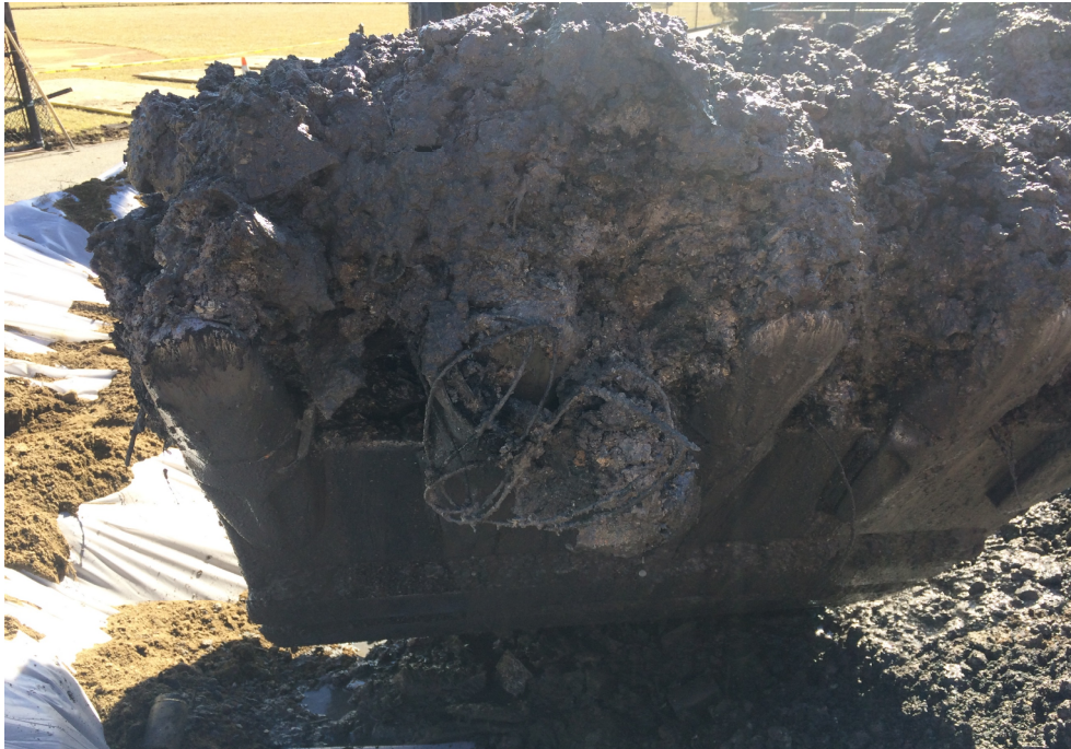
-Bucket of waste fill material from approximately 13' bgs
