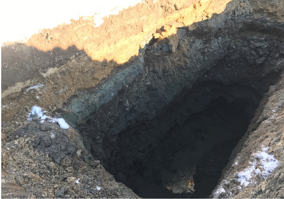
-Exposed north sidewall with groundwater at approximately 9.5' bgs
