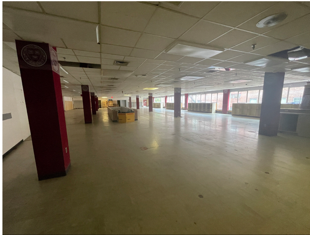
Existing Conditions - Third Floor
