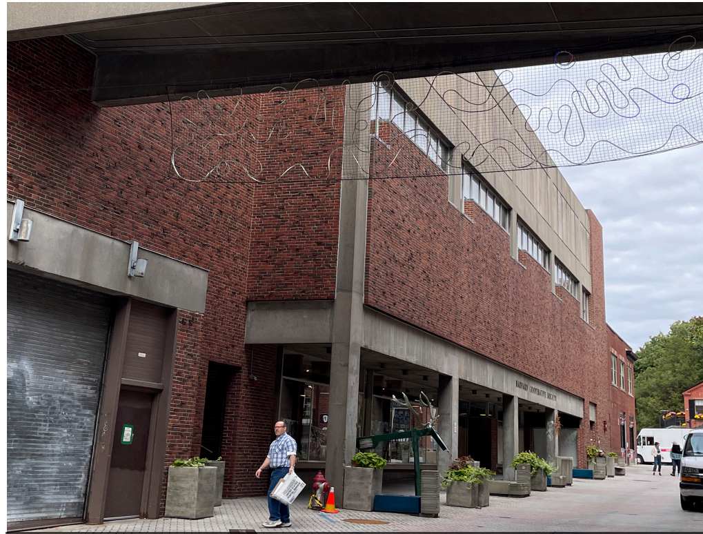
Existing Conditions - Exterior
