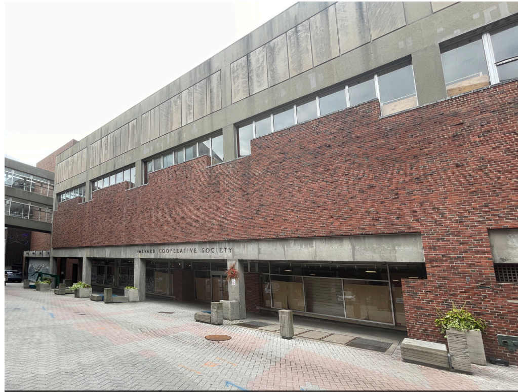
Existing Conditions - Exterior
