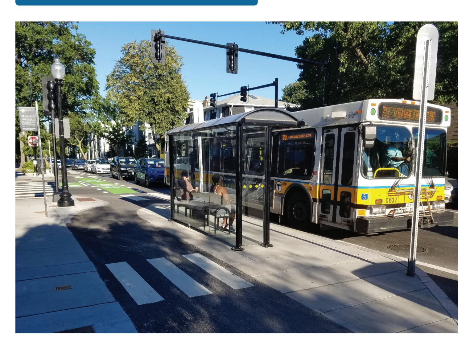
"Floating" bus stops reduce conflicts between bikes and buses while enabling buses to stop in-lane (rather than pulling in and out of a bus stop) to improve transit speeds and reliability.
