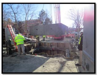
Phase two (2) consists of installing the concrete sections of the storage tank. The storage tank work has begun and will continue until the beginning of June. The concrete section installation will require a series of excavations and placement of pre-cast concrete structures using a large crane. This work may cause you to feel vibrations and an engineer will be on site to measure and monitor these vibrations.
