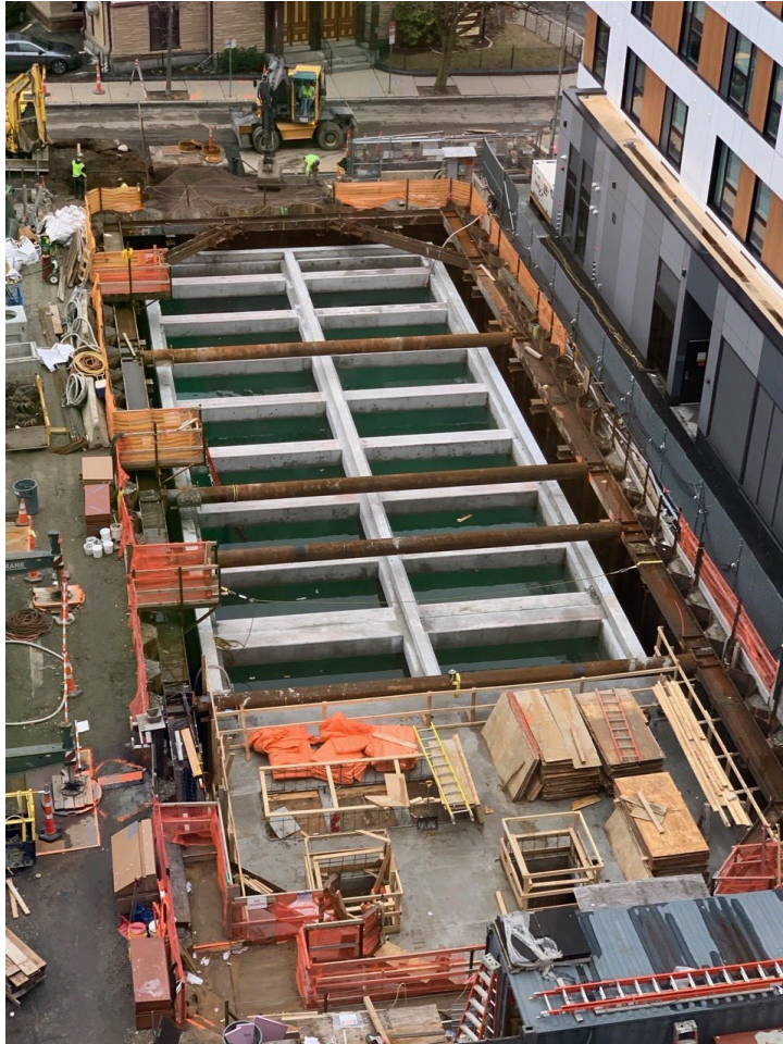
PL6 Tank w/ Braced SOE
