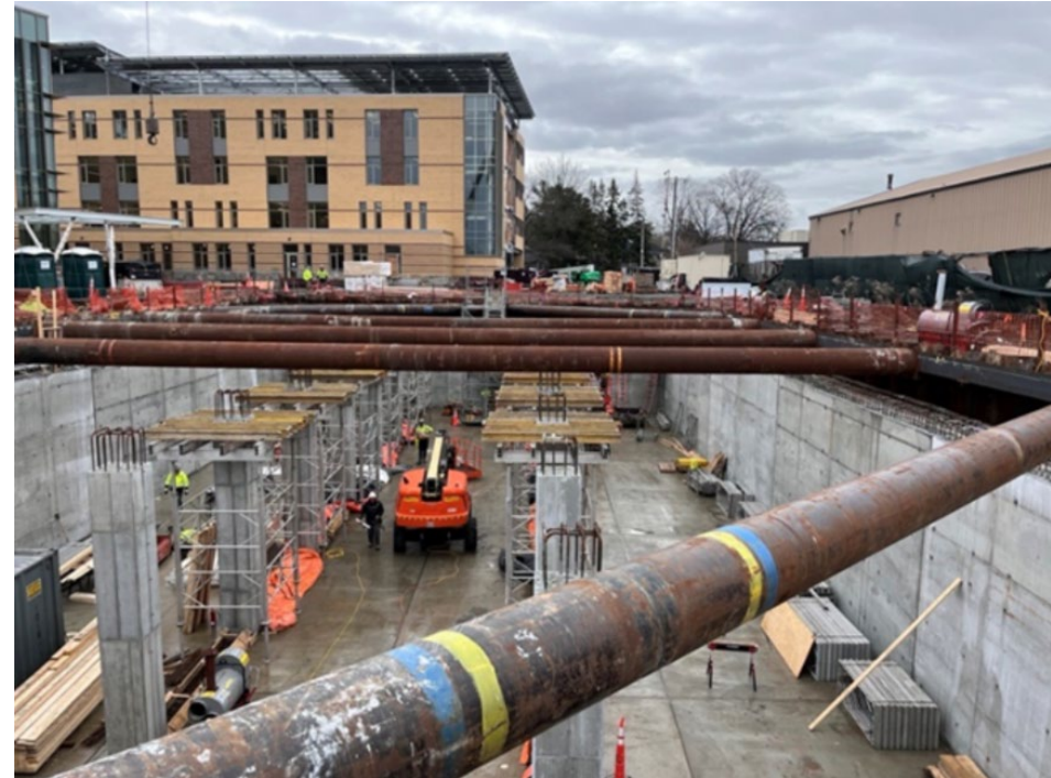
Tobin Tank w/ Braced SOE
