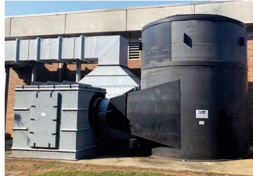
Odor Control Alternative – Radial Pure Air Model 0810
