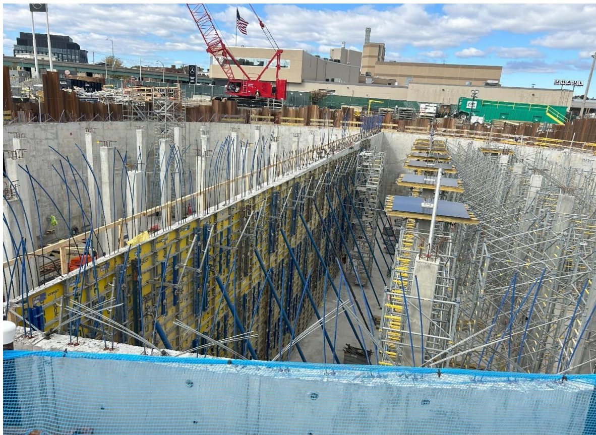
Figure 3-17. AWWA D115 Tendon-Prestressed Cast-in-Place Circular Tank
