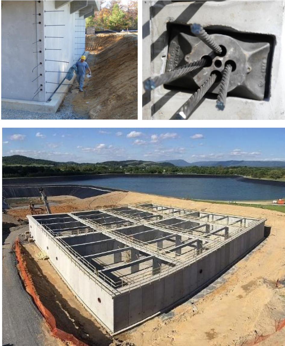
Figure 3-16. AWWA D115 Tendon-Prestressed Precast Rectangular Tank
