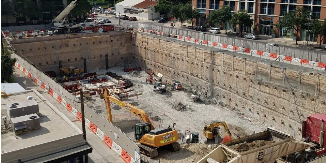
Figure 3-14. Excavated Diaphragm Wall with Tieback Anchors (Keller)
