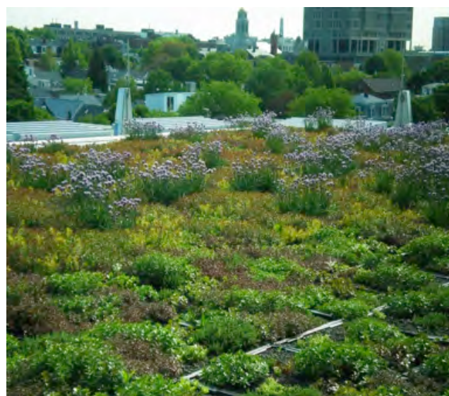
(top) Broadway: July 10, 2010. (middle) Constructed wetland, North Point (bottom) Green Roof at the Robert W. Healy Public Safety Facility in East Cambridge.
