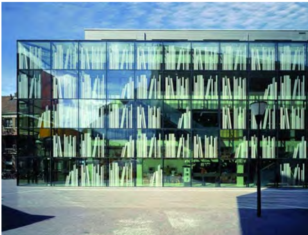
People in the community expressed interest in a new library that would be much more visible than the existing branch library. This example is very glassy, and makes its presence as a library very visible.
