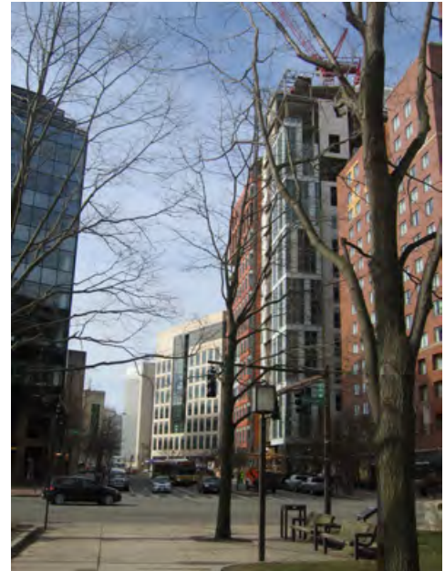
Expansion of the Broad Institute along Ames St shown in the middle. The existing Broad building is to the left of the new building.
