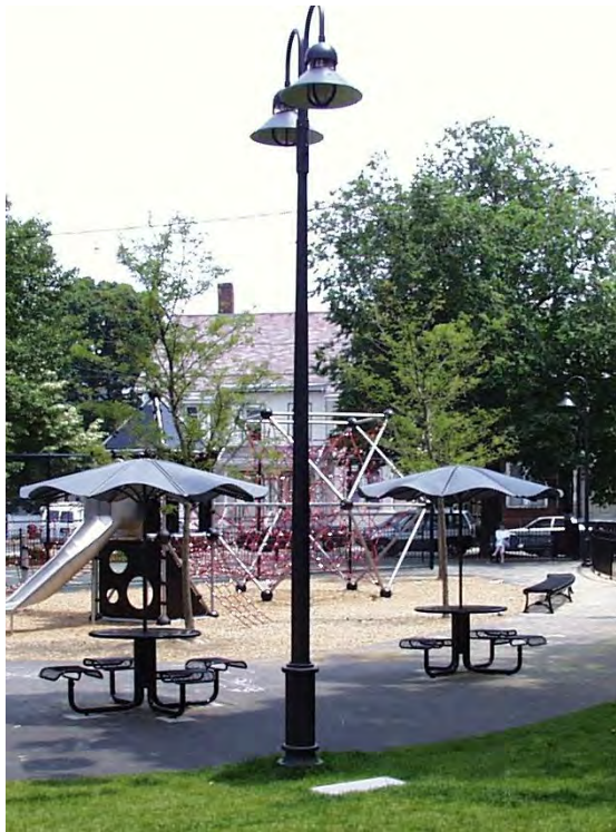
Sheperds Crook fixture used in Cambridge parks – in single and double configuration
