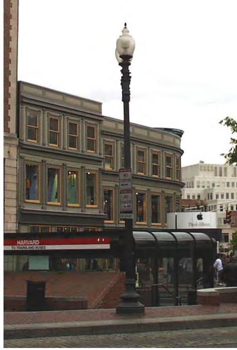
Pedestrian scale Acorn post-top fixtures – Harvard Square
