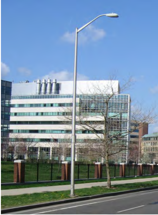
Cobraheads are the most common light fixture in the City
