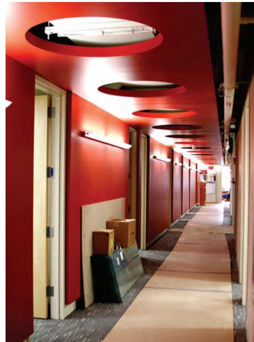
Renovation progress in Building E18
