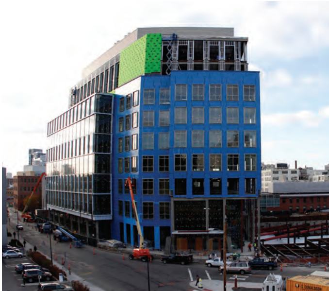
Construction at 610 Main Street
