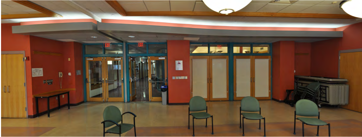
Fig. 403 - View of entry area, lowered ceiling/fluorescent cove light & partition track
