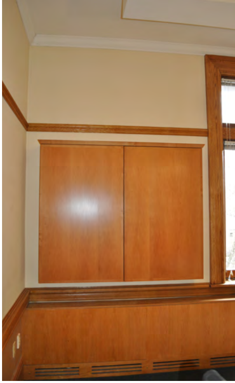
Fig. 302 - Existing Smartboard & Cabinet
