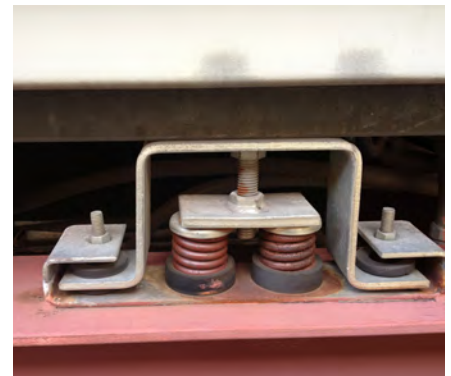
Fig. 416 - Rooftop equipment vibration isolator
