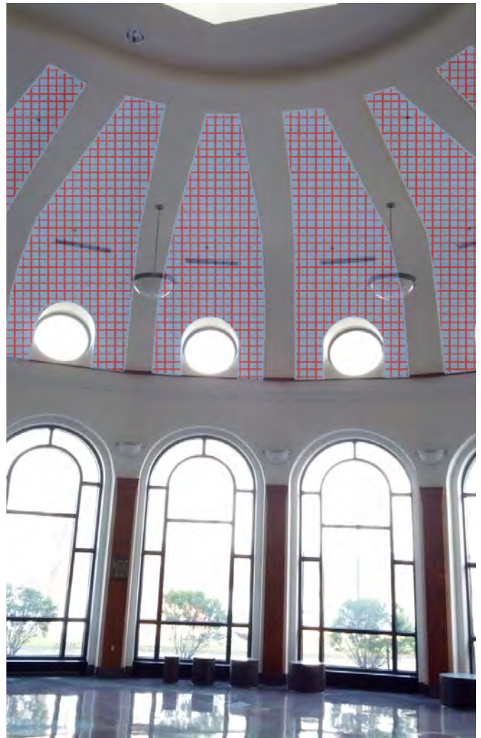
Fig. 605 - Curved ceiling coffers
