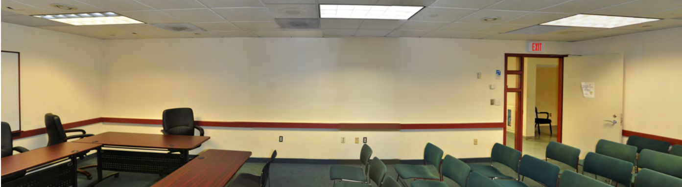
Fig. 701 - Existing conditions (note “scalloping” from existing fixtures)
