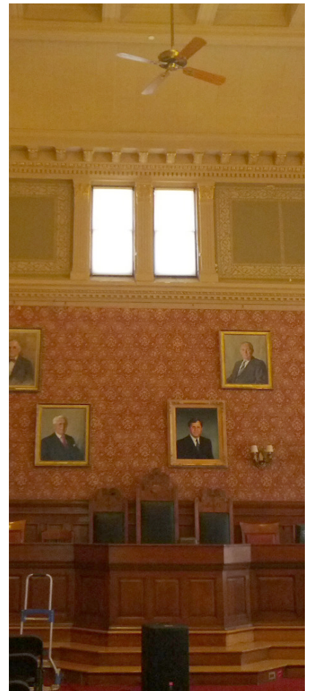
Fig. 118 - Glare from existing windows
