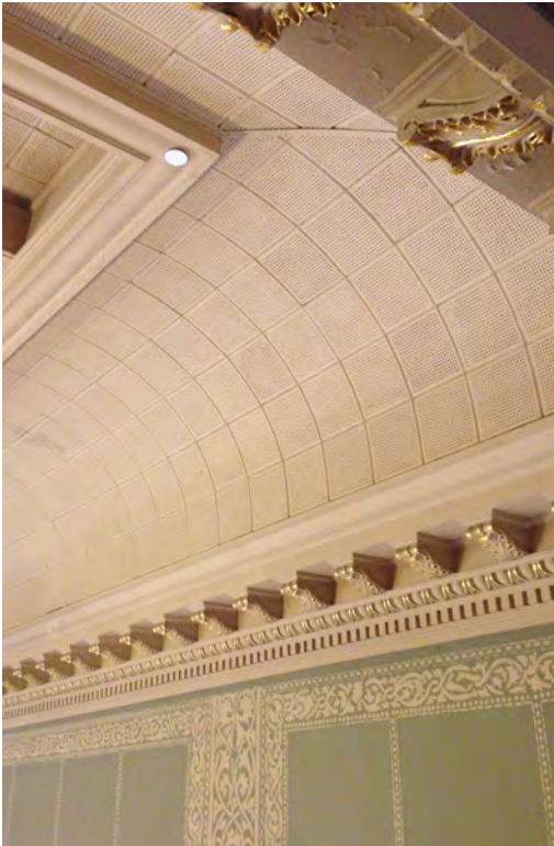
Fig. 104 - Existing Acoustic Tile
