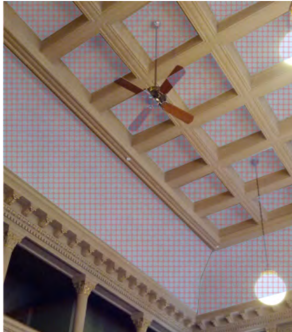
Hatched area indicating existing acoustical ceiling tiles
