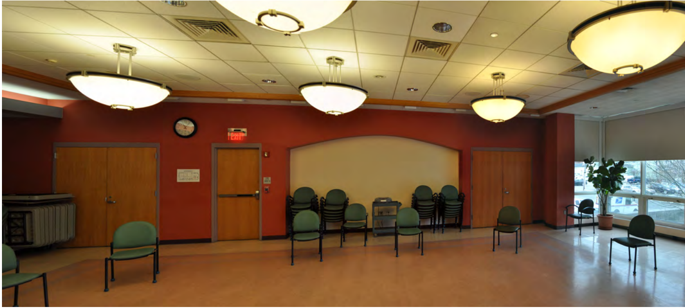
Fig. 404 - View of existing pendant fixtures, ceiling diffusers and glazed wall
