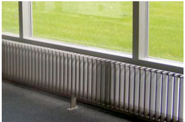
Fig. 127 - Proposed Runtal RS-2 Radiators
