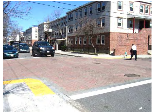
Raised crossings at intersections were installed as part of improvements to Windsor Street.
