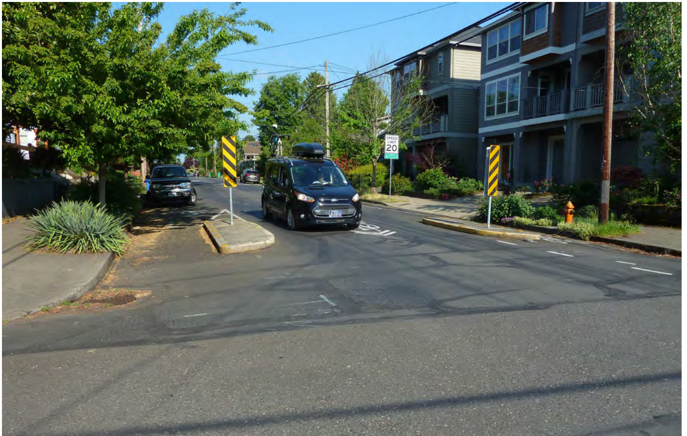
Figure G.5: Photo of a Pinch Point with Bike Cut-throughs
