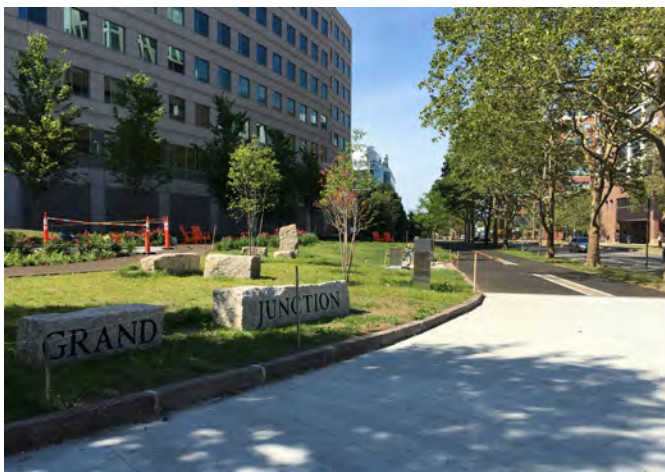
The first portion of the Grand Junction multi-use path was constructed by the Cambridge Redevelopment Authority.
