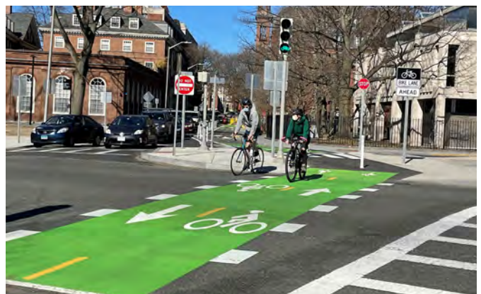
Harvard constructed the bicycle facilities along the Quincy-DeWolfe corridor, to help people travel to and from the Charles River to Harvard Square and Harvard Yard.
