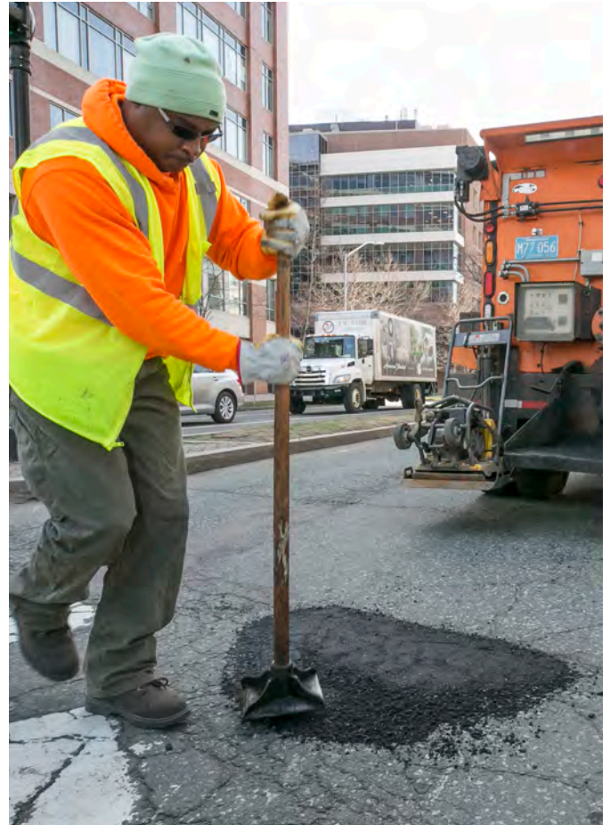
From restriping to filling potholes, taking care of roadways and bike facilities is critical to maintaining safe conditions for biking in Cambridge.
