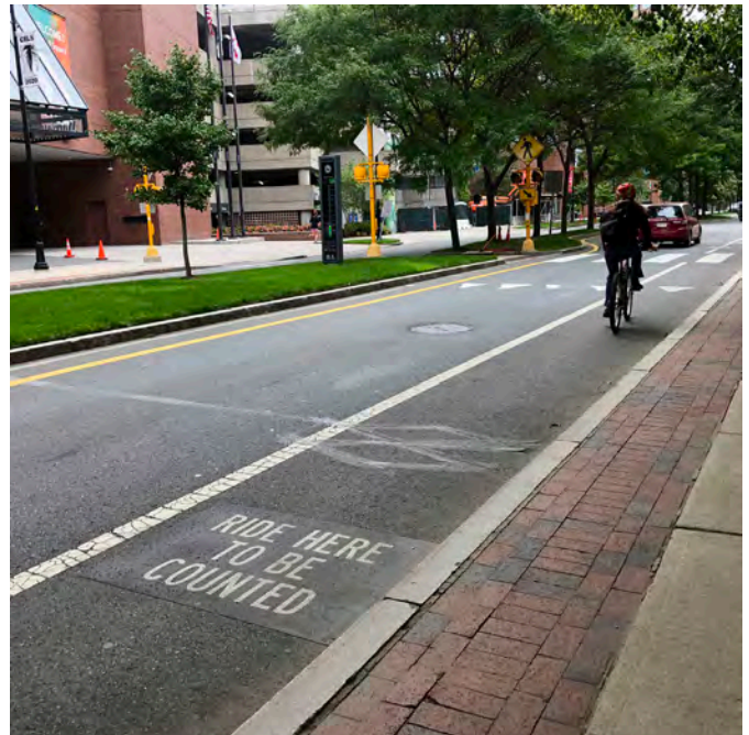
The City added directional information on the pavement as one way to communicate the need for a bicycle to track over the loop in order to trigger the Eco-Totem counter.
