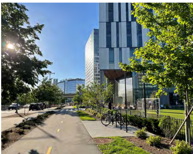
Connected paths were constructed in North Point as part of EF's campus expansion.
