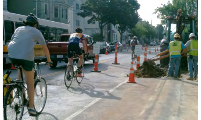
Construction zone featuring temporary bike lane.
