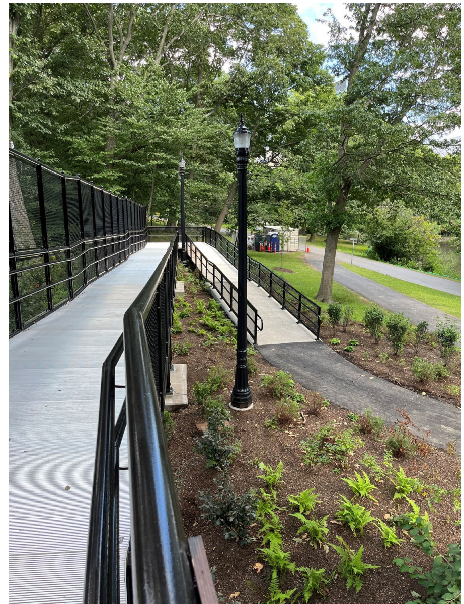
Carlton Street Footbridge Brookline, MA
