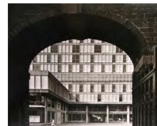
Left: Arcade: Sert's original idea is one of an open arcade linking three open spaces
