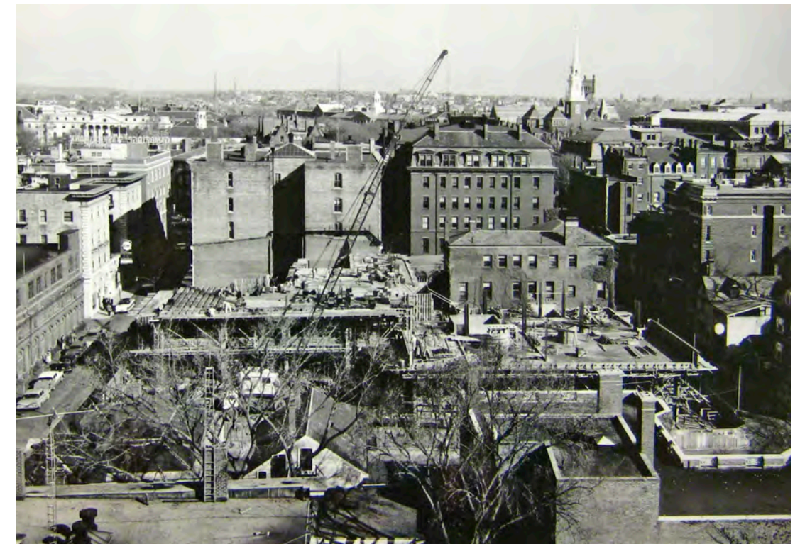
Phase I construction, looking north from the Malkin Athletic Center, circa 1960
