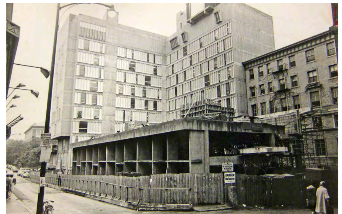
Phase 1B construction of shops on Holyoke Street, circa 1963, Phase 1A is completed in the background
