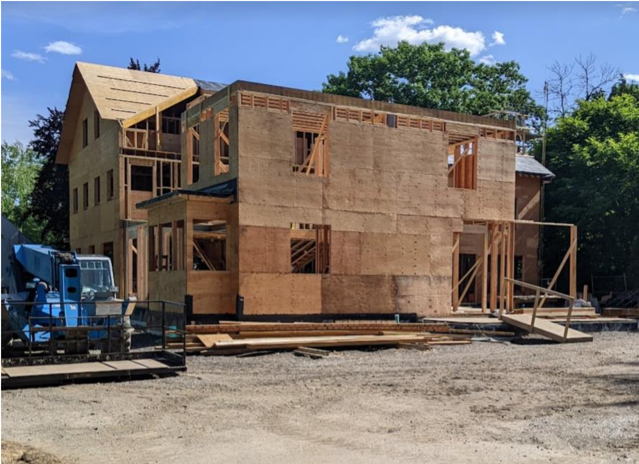
12 Lake View Avenue after removal of nearly all original material, June 22, 2022
