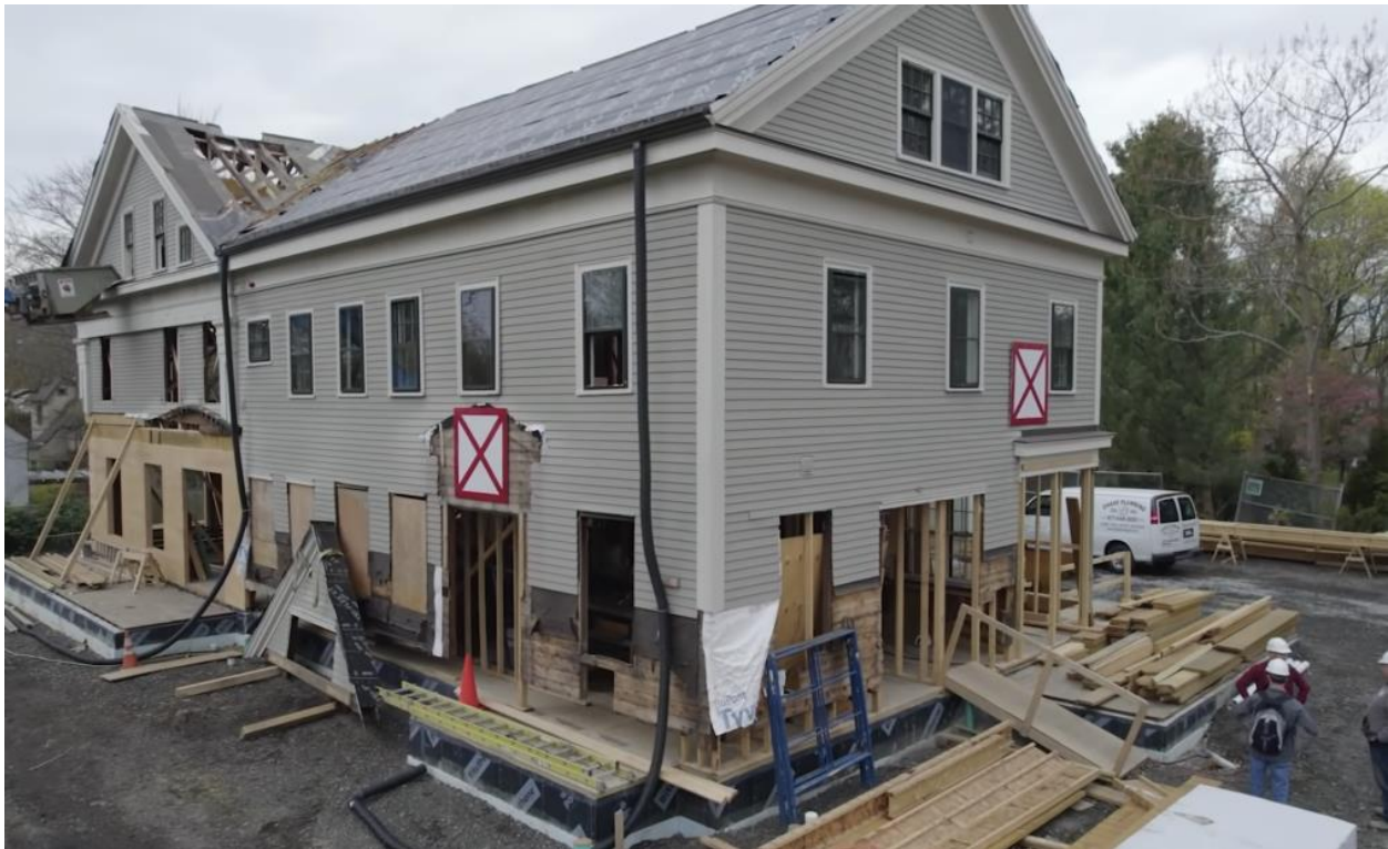
12 Lake View Avenue lowered on its new foundation, with original framing and exterior still in place, Spring 2022. Screenshot, The Bridge podcast.
